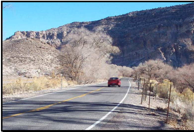
State Route 317, Lincoln County
