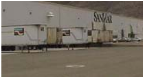
Tahoe Reno Industrial Park
