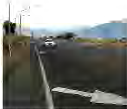
Acceleration and deceleration lanes allow drivers to slow down to enter a side street or speed up before entering moving traffic.
