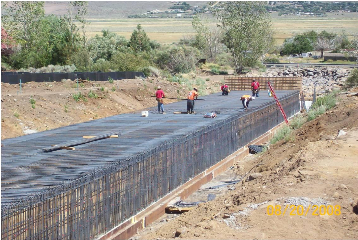
Reinforced Concrete Box Stakeout
