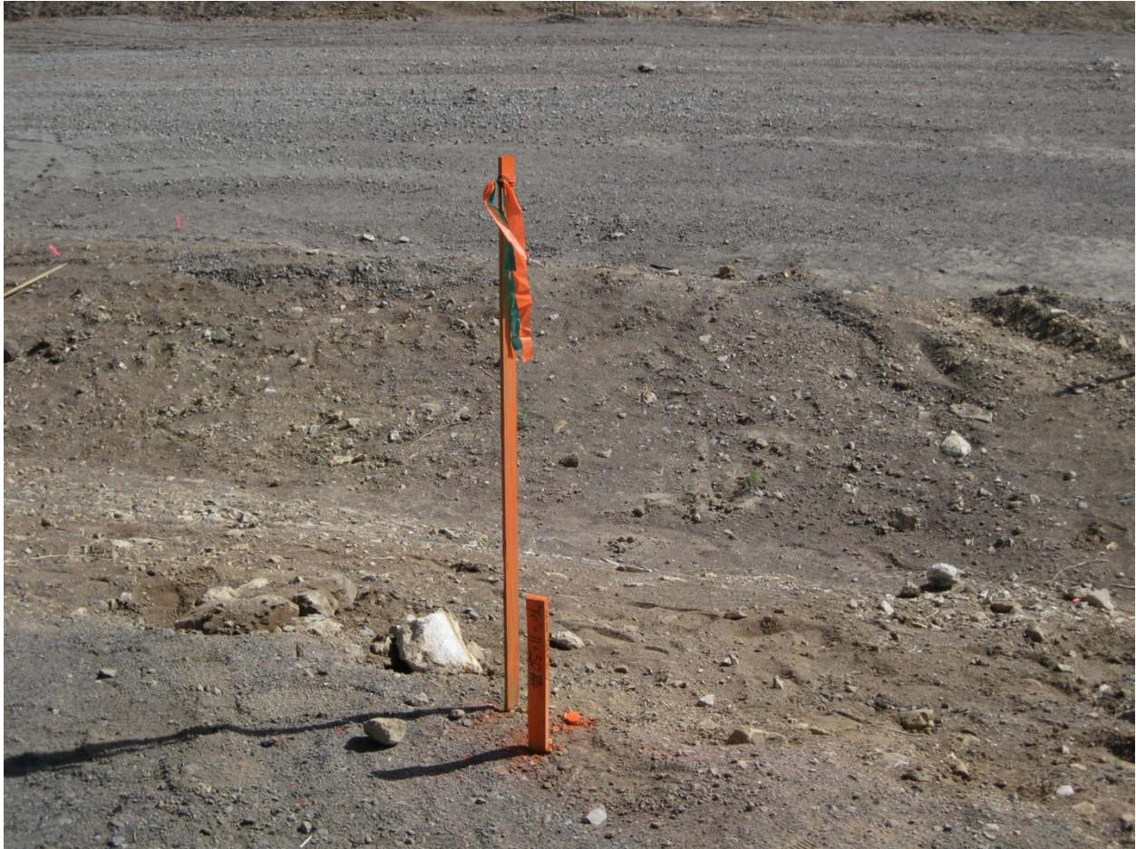
Slope Stake with Guard Lath
