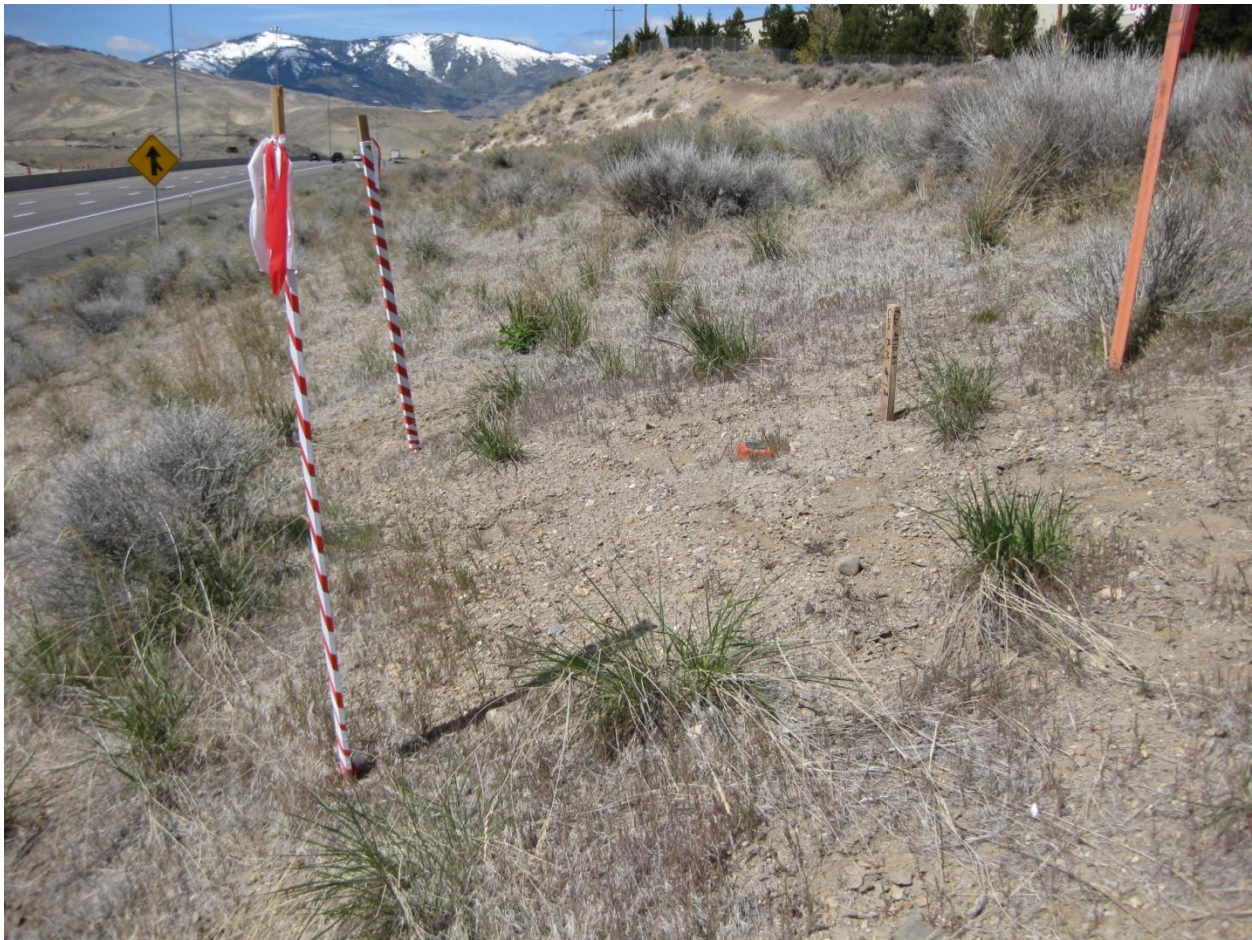
Construction Control Feno Monument
