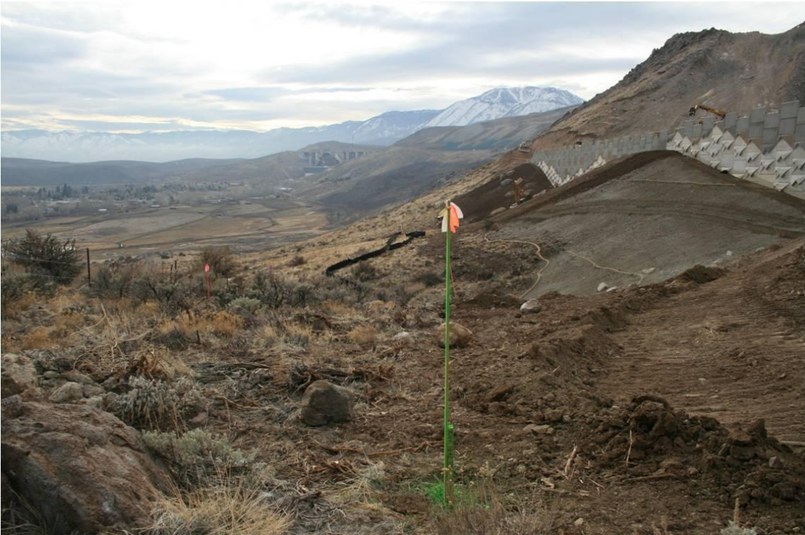
Slope Stake on the I-580 Project (Contract 3292)
