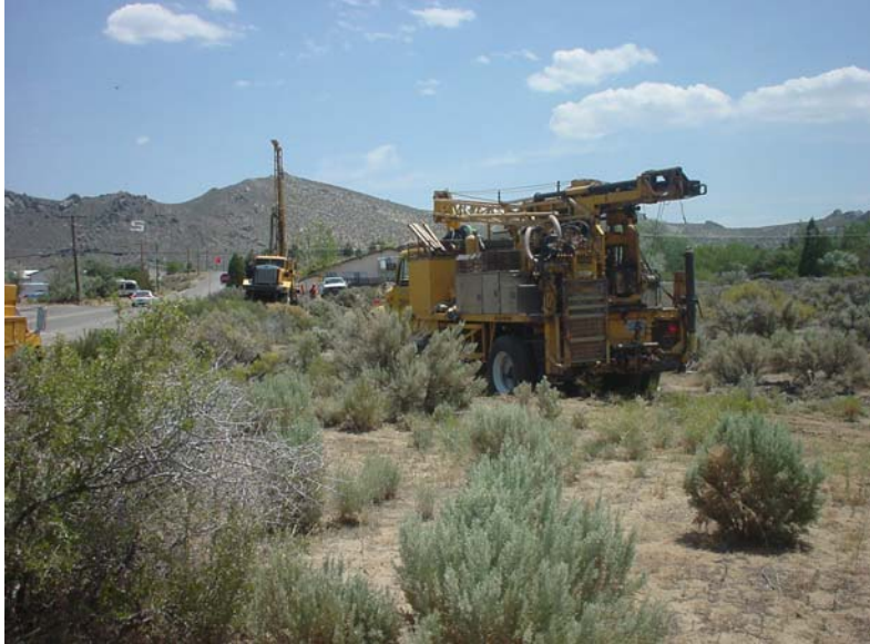
Photo 2. Clearview Drive: Looking East toward S. Edmonds Drive.
