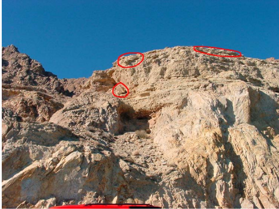
Fig 3. Milepost 63.2 showing loose rock and alluvium overhang.
