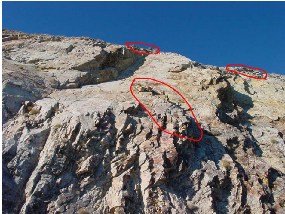
Fig 8. Milepost 63.38 showing highly fractured rock and soil overhang. Note highly fractured bedrock in foreground with many loose wedges.
