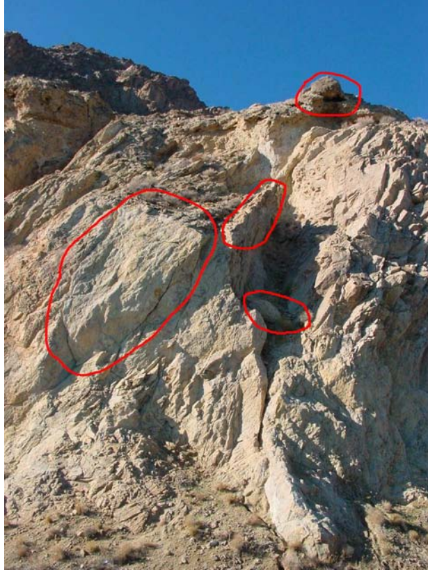
Fig 21. Milepost 63.85 showing large fractured bedrock wedge, overhanging bedrock, perched boulder and cemented soil overhang.
