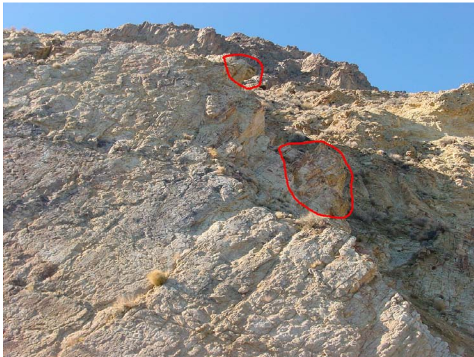
Fig 20. Milepost 63.83 showing large, overhanging, fractured bedrock.
