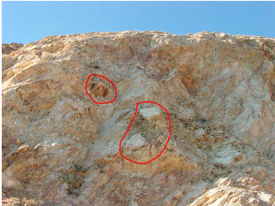
Fig 10. Milepost 63.50 showing larger blocks of fractured rock.
