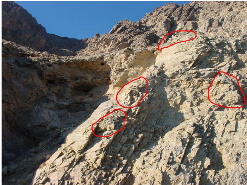
Fig 24. Milepost 63.93 showing intensely fracture bedrock wedges and soil overhang.
