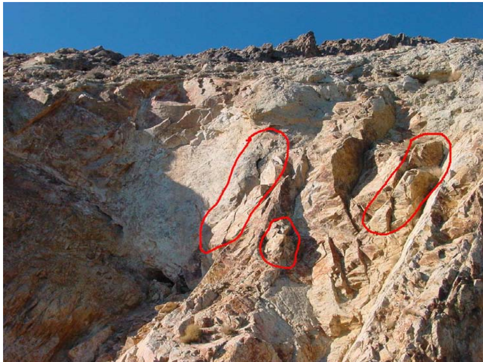
Fig 18. Milepost 63.75 showing open fractures in rock creating unstable wedges of rock.
