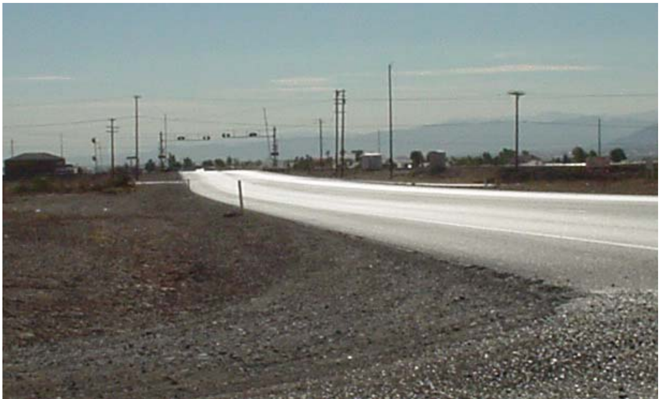
Photo 1. SR 160 (Blue Diamond Road): Looking West toward UPRR at-grade Crossing
