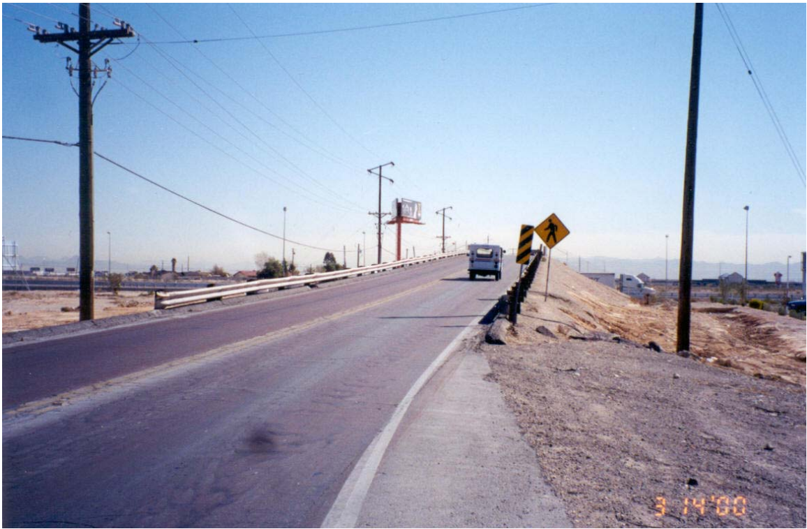
Photo 1. Original structure, looking to the west.
