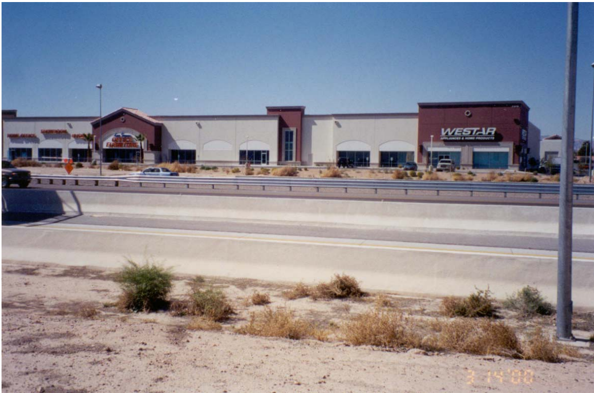
Photo 2. Buildings to the south west of the current structure.
