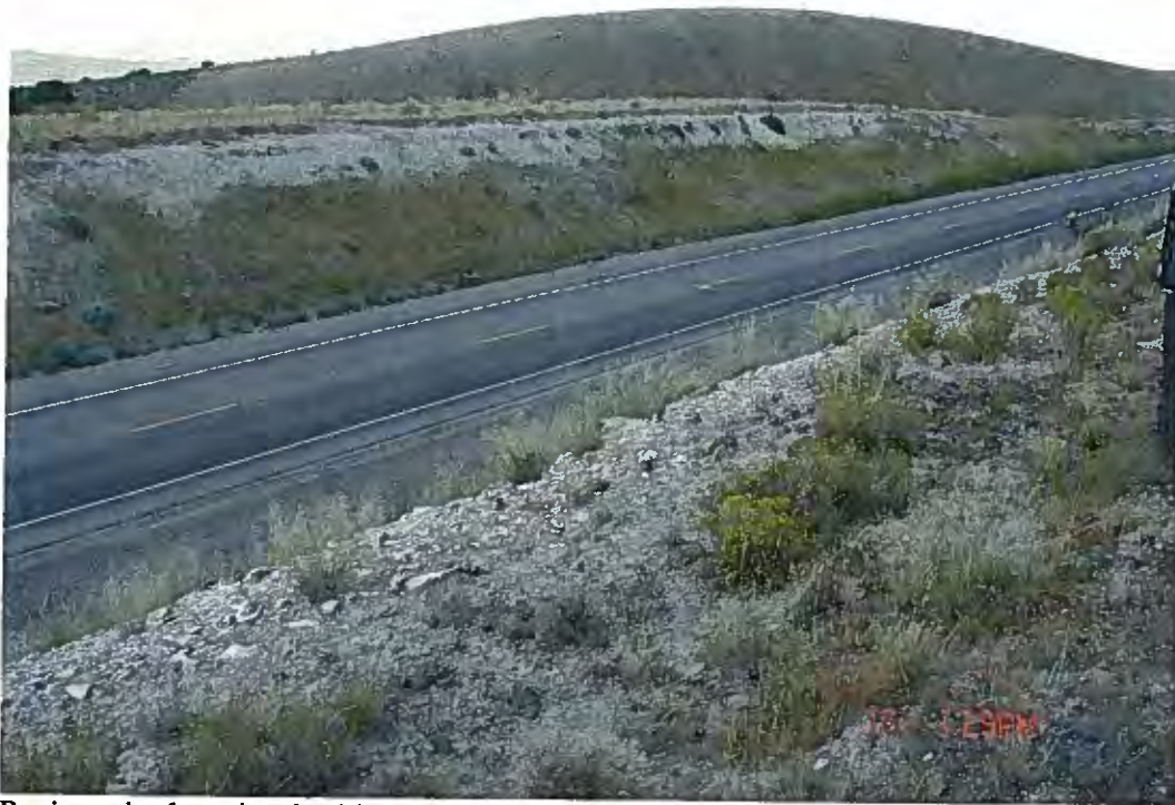
Project site location looking south east with Windermere Hills in the background.
