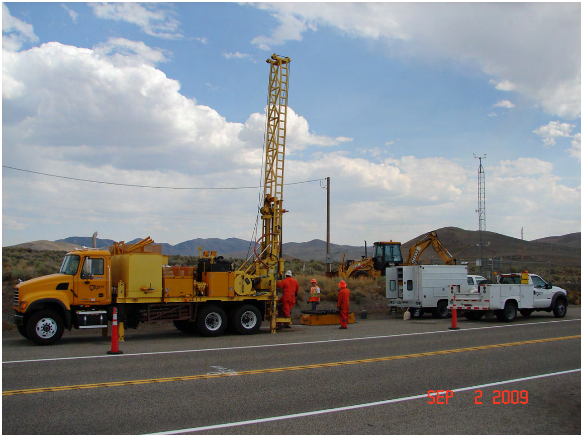
Photo 2. Drill Rig Setting Up on Borehole OC-4.
