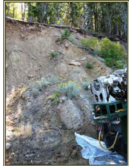
Figure 3 – Slope 21, West End
