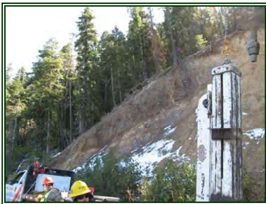
Figure 4 – Slope 27, East End
