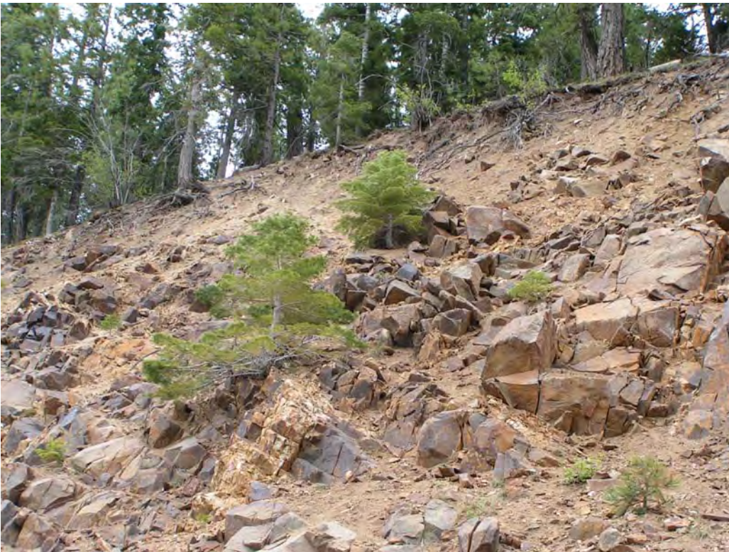
Portions of Slope 27 have some mature vegetation starting to grow
