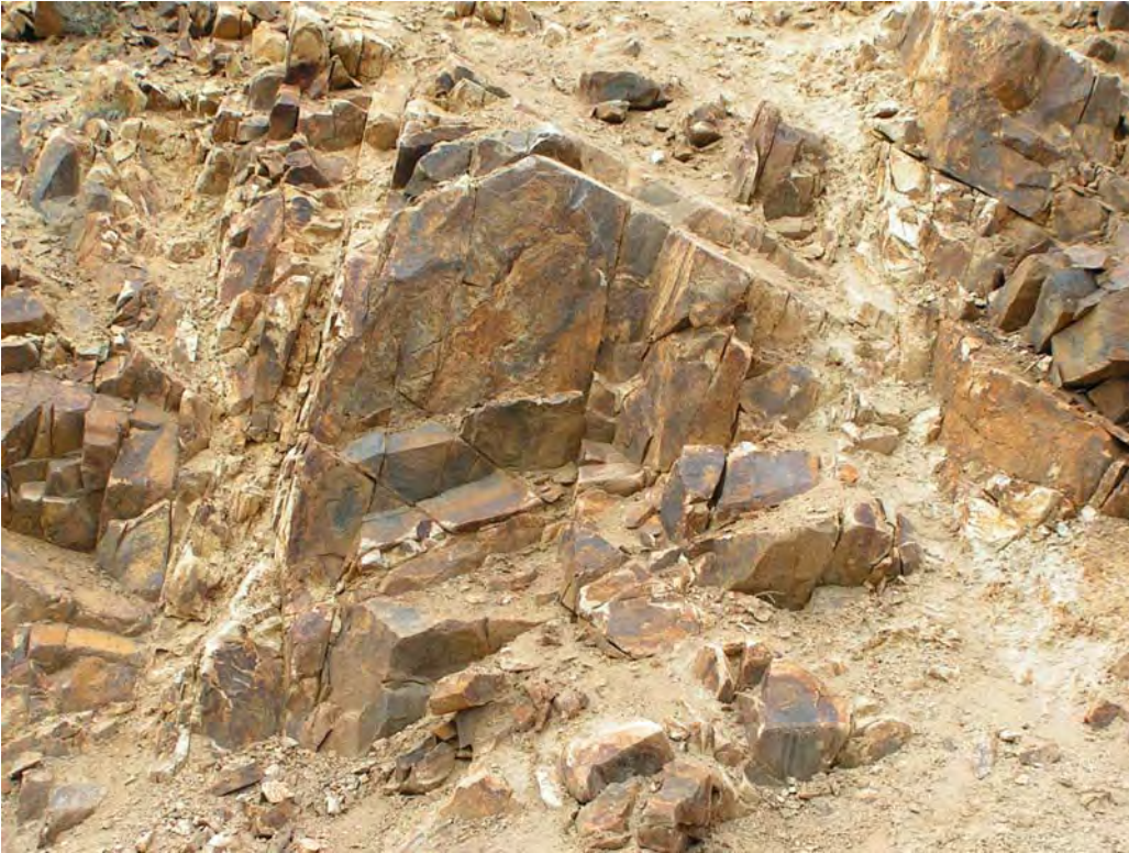
Slope 27 exhibits wedge, sliding and topple failure fracture sequences
