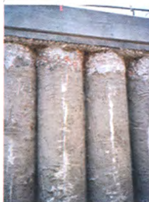
Completed Tangent Pile Wall
