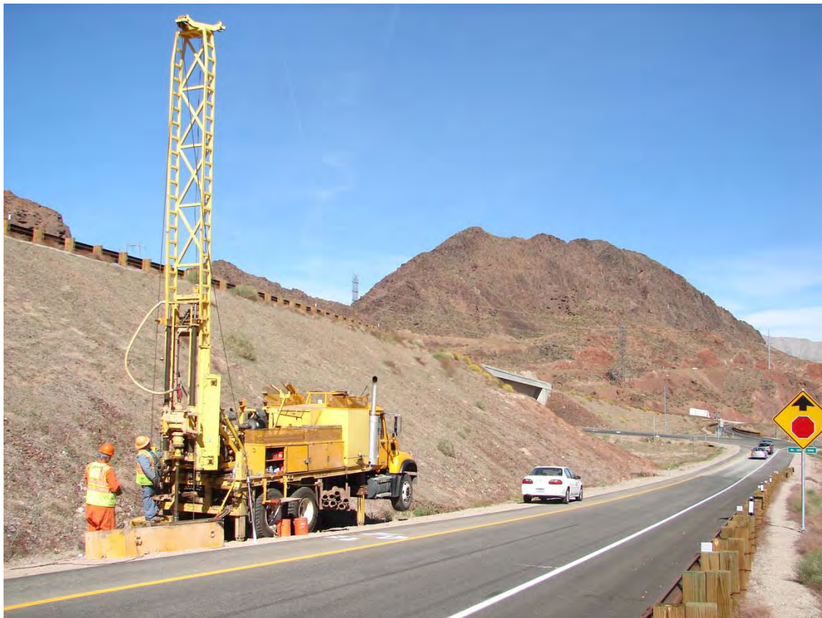
Photo 5. Drill rig set up on Borehole BCR-4
