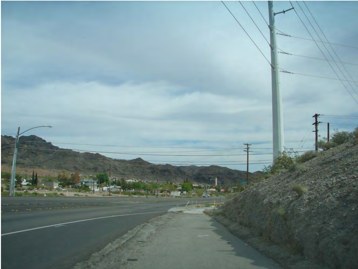
Photo 9. Existing cut slope at Colorado Street
