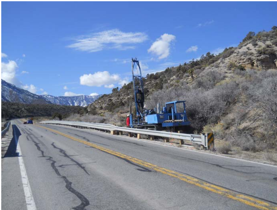
YA-14 - Kyle Canyon at MP 7.00 Near Single Box Culvert Inlet
