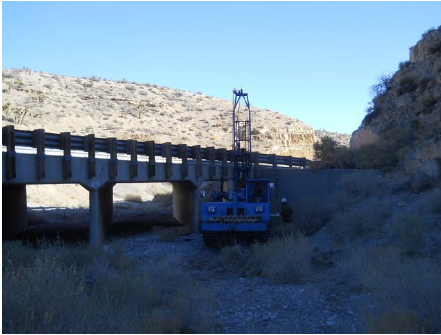
YA-13 - Kyle Canyon at MP 11.00 Triple Box Culvert Inlet
