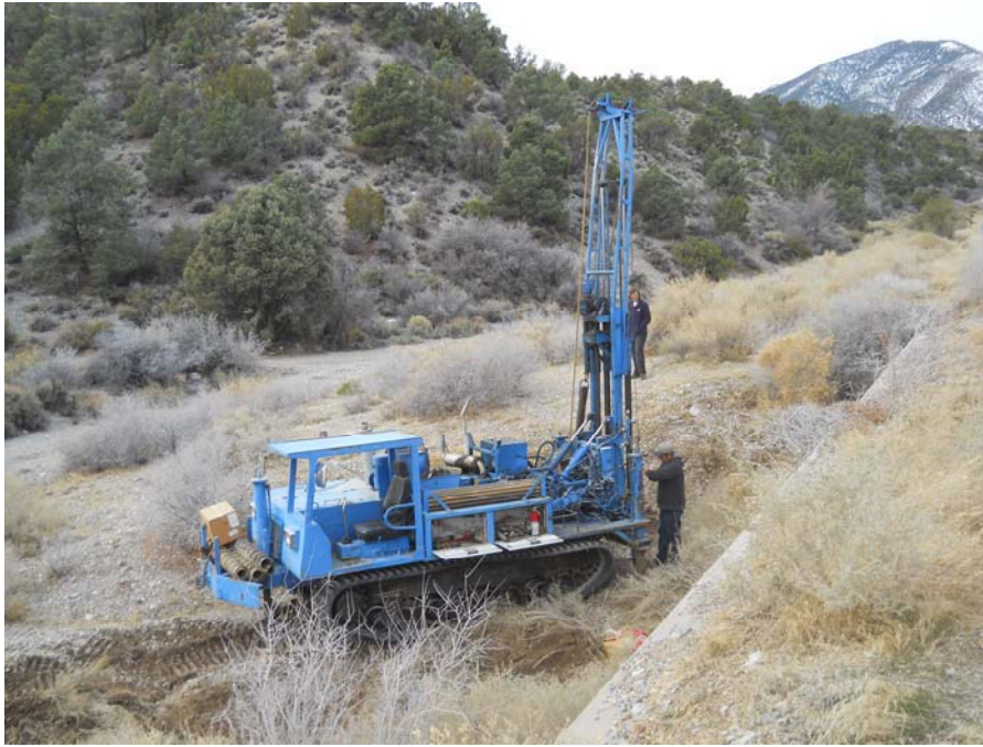
YA-09 - Kyle Canyon at MP 7.00 Double Box Culvert Outlet
