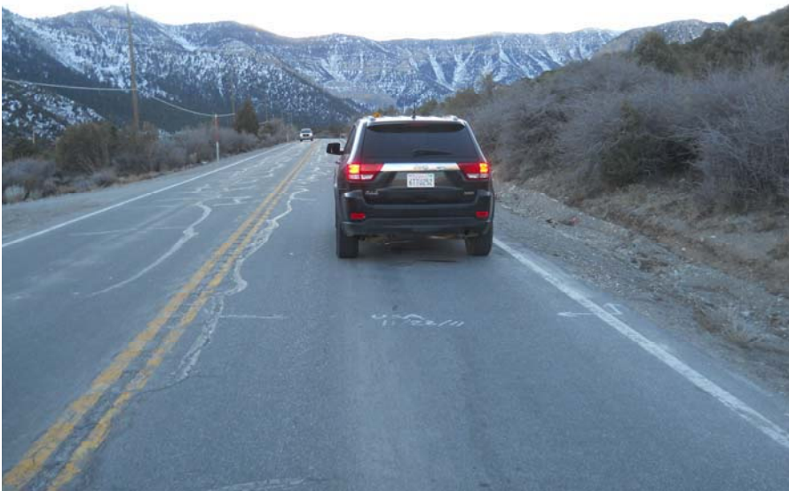
YA-04 – Kyle West Roundabout – Westbound
