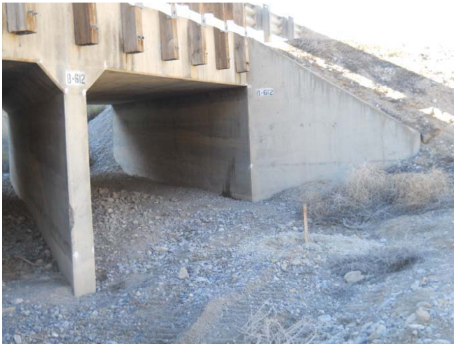
YA-12 - Kyle Canyon at MP 11.00 Triple Box Culvert Outlet
