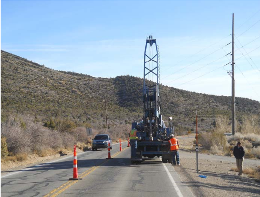
YA-01 – Kyle West Roundabout – Eastbound
