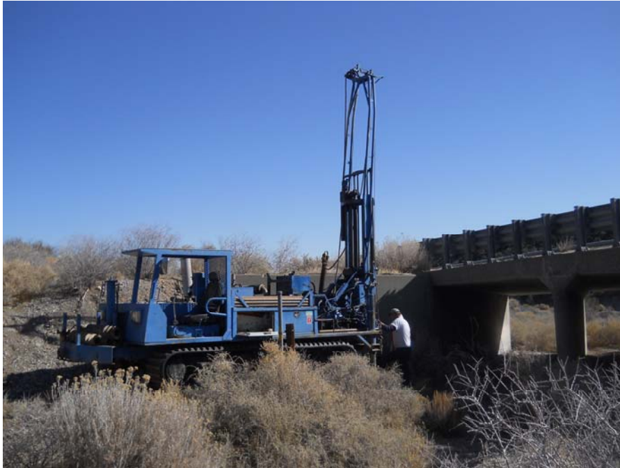
YA-11 - Kyle Canyon at MP 7.00 Double Box Culvert Inlet
