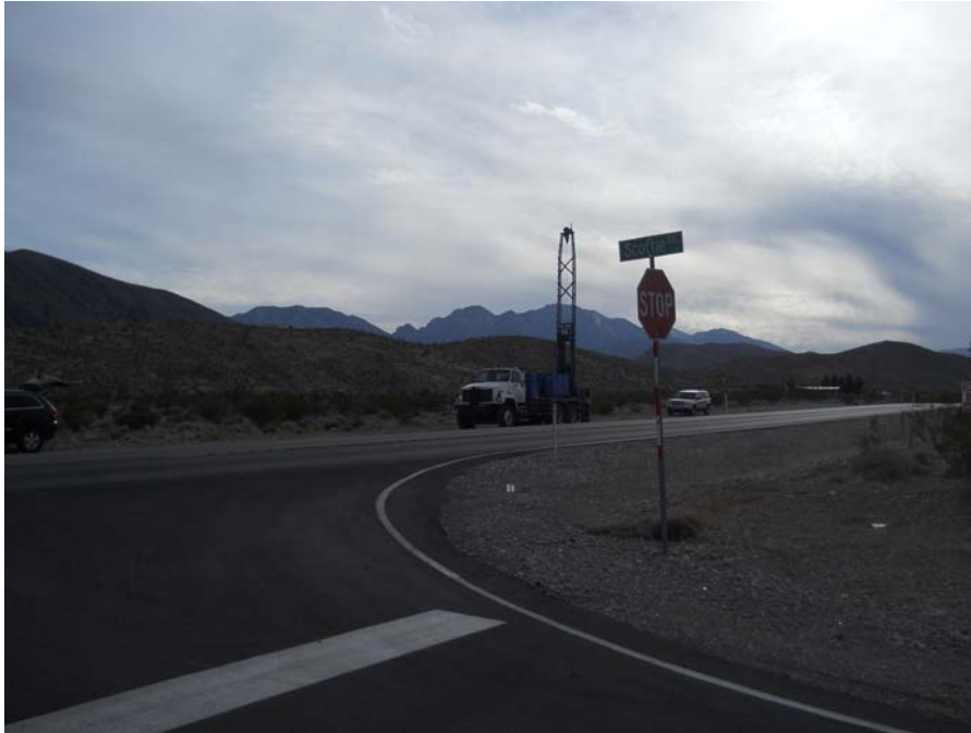
YA-07 – Kyle Canyon Road near Scottie Road – Eastbound
