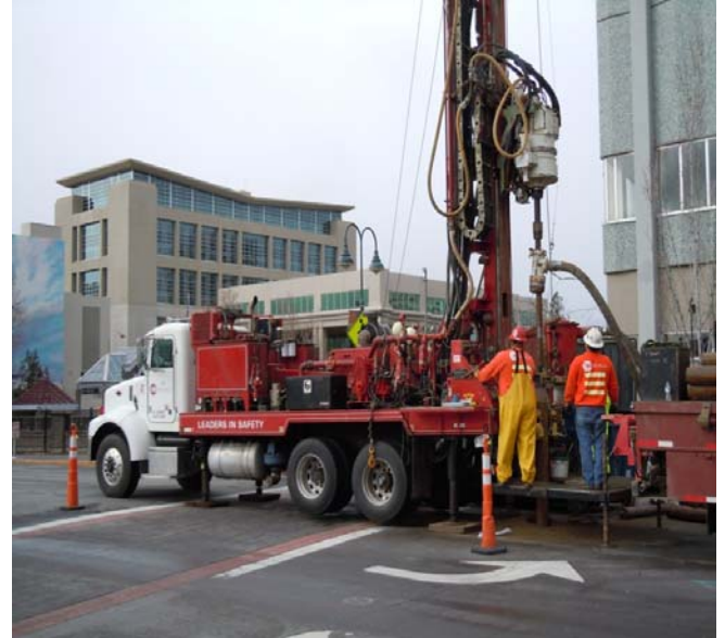
VSB North Abutment Exploration Drilling
