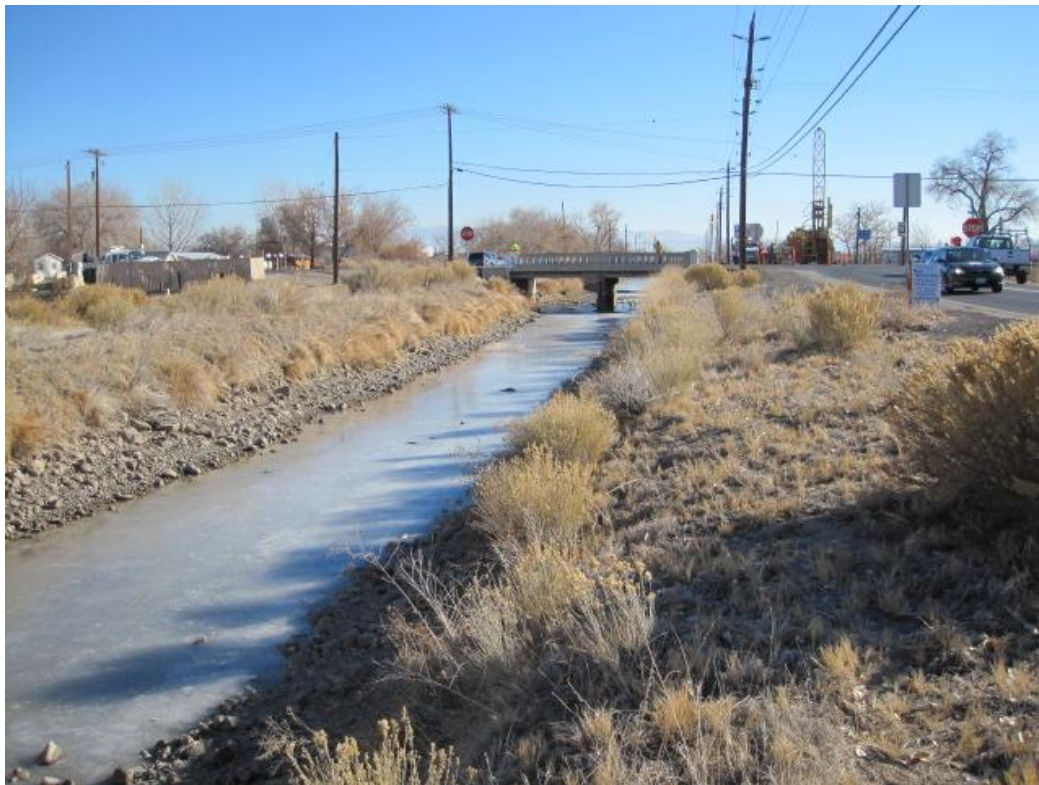
Photo 1. Looking East (downstream) towards Bridge B-100.
