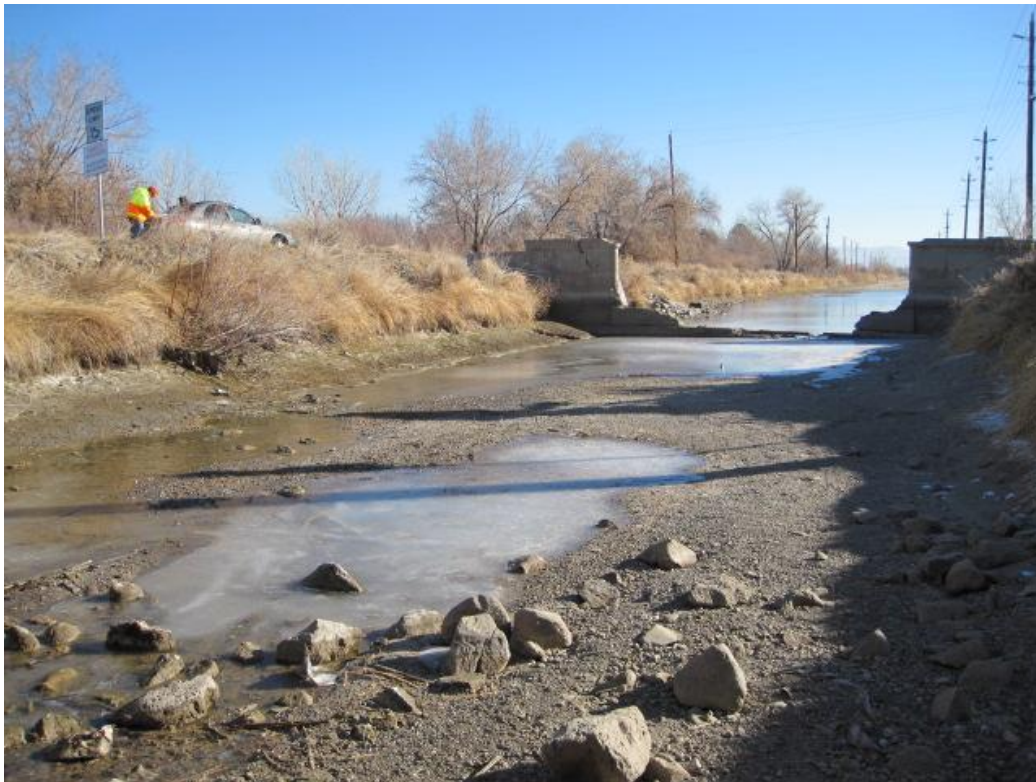
Photo 3. Looking East (downstream) towards the weir from Bridge B-100.
