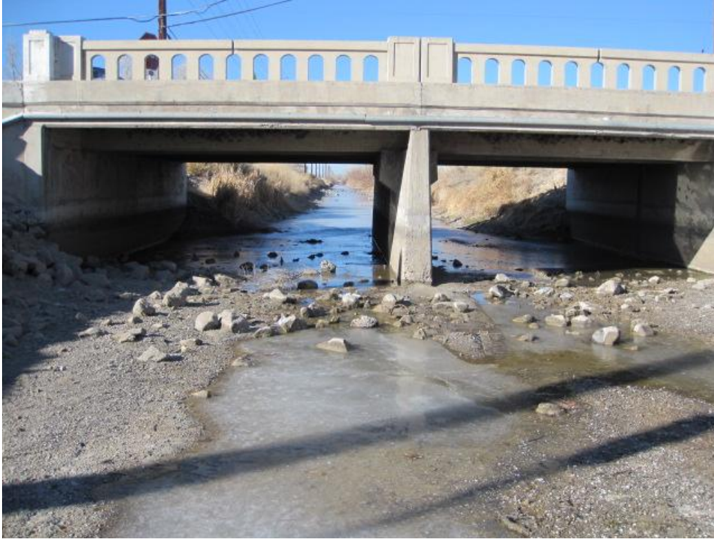
Photo 2. Looking West (upstream) at Bridge B-100.
