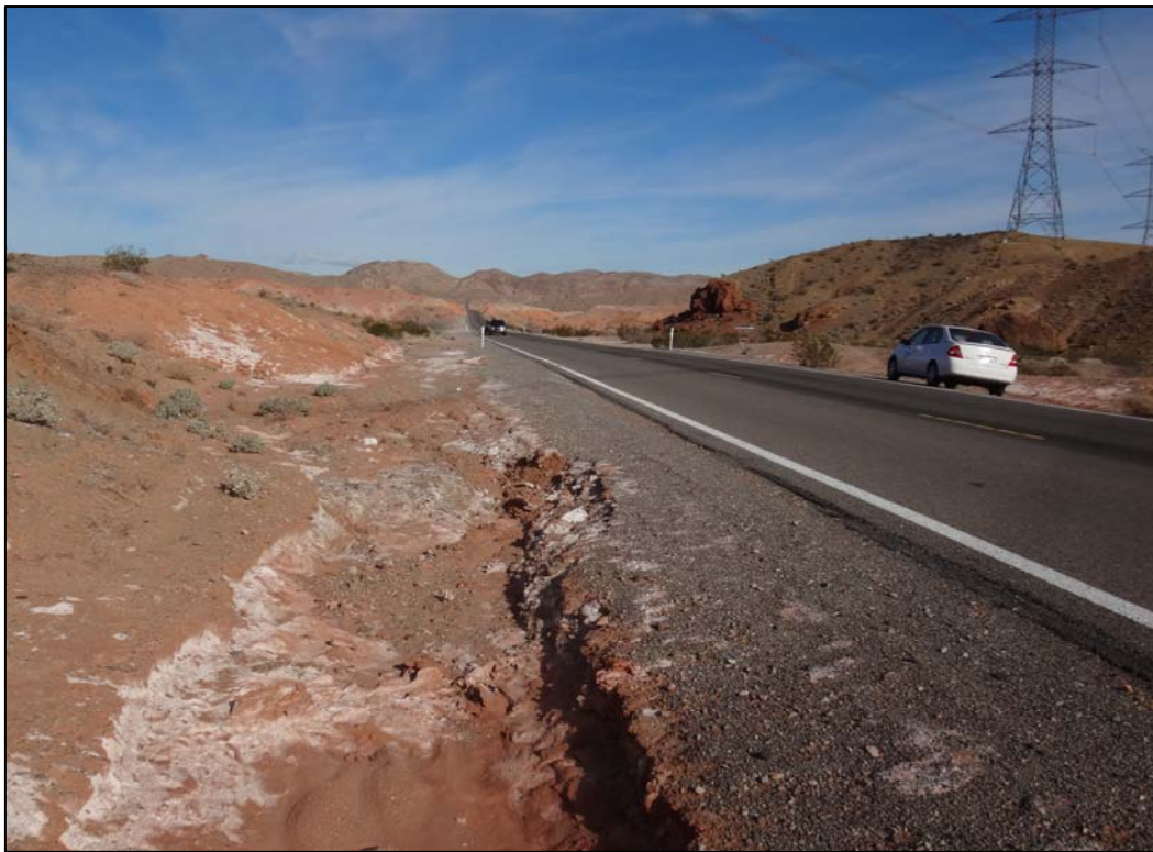
Picture 1: Looking North along SR147
