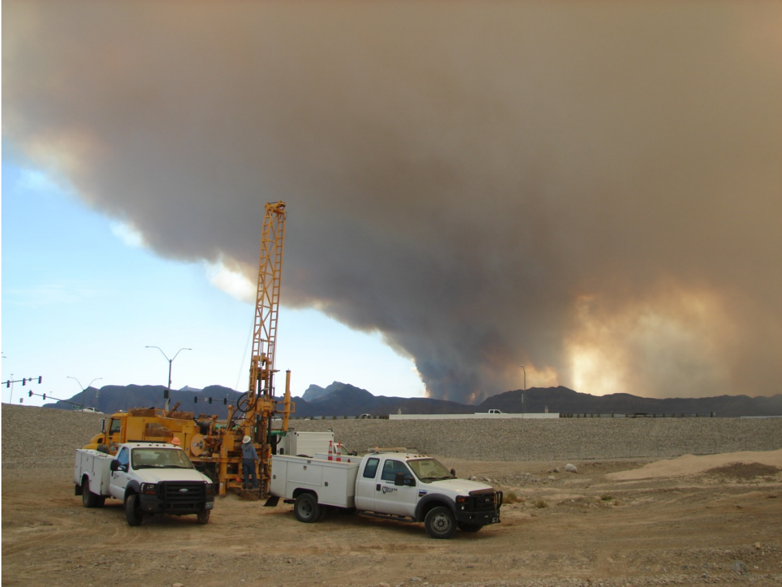
Photo 3. Drill Rig Set Up on Borehole BI-29 (with Carpenter fire in background)
