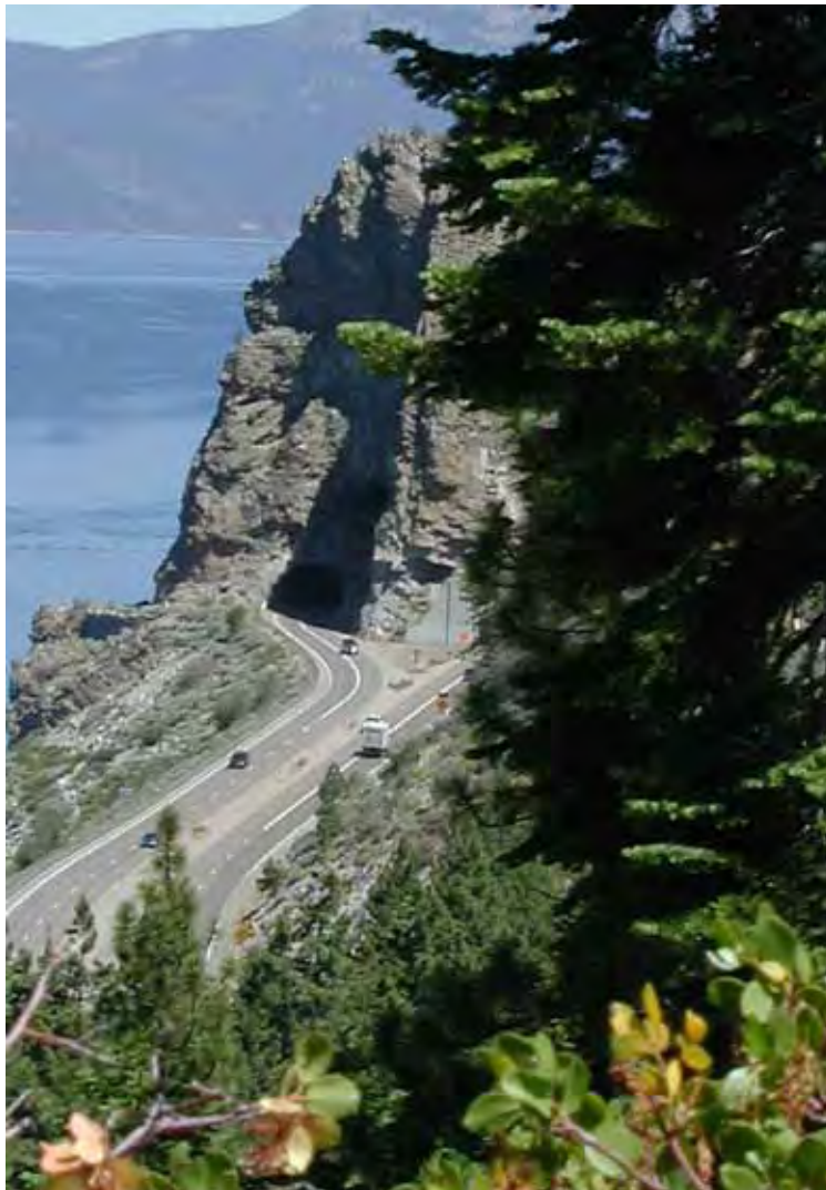
US 50 Cave Rock Tunnel, Lake Tahoe
