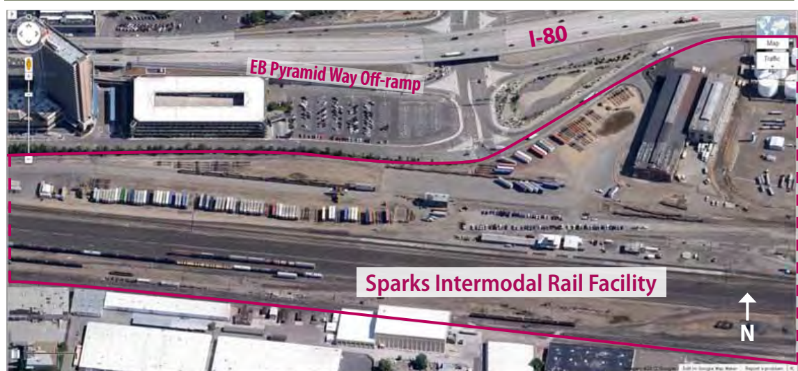
Figure 26. Sparks Intermodal Rail Facility
