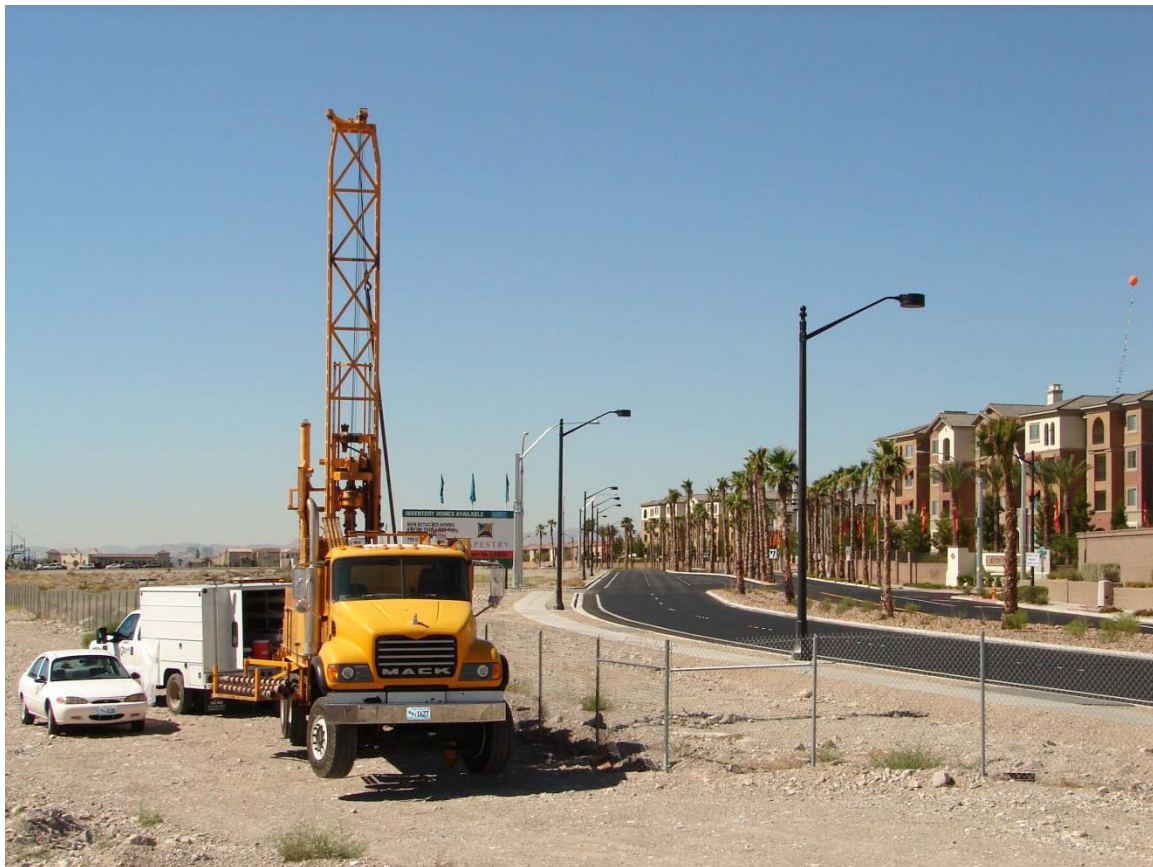
Photo 3. Drill Rig Set Up on Borehole ASW-17
