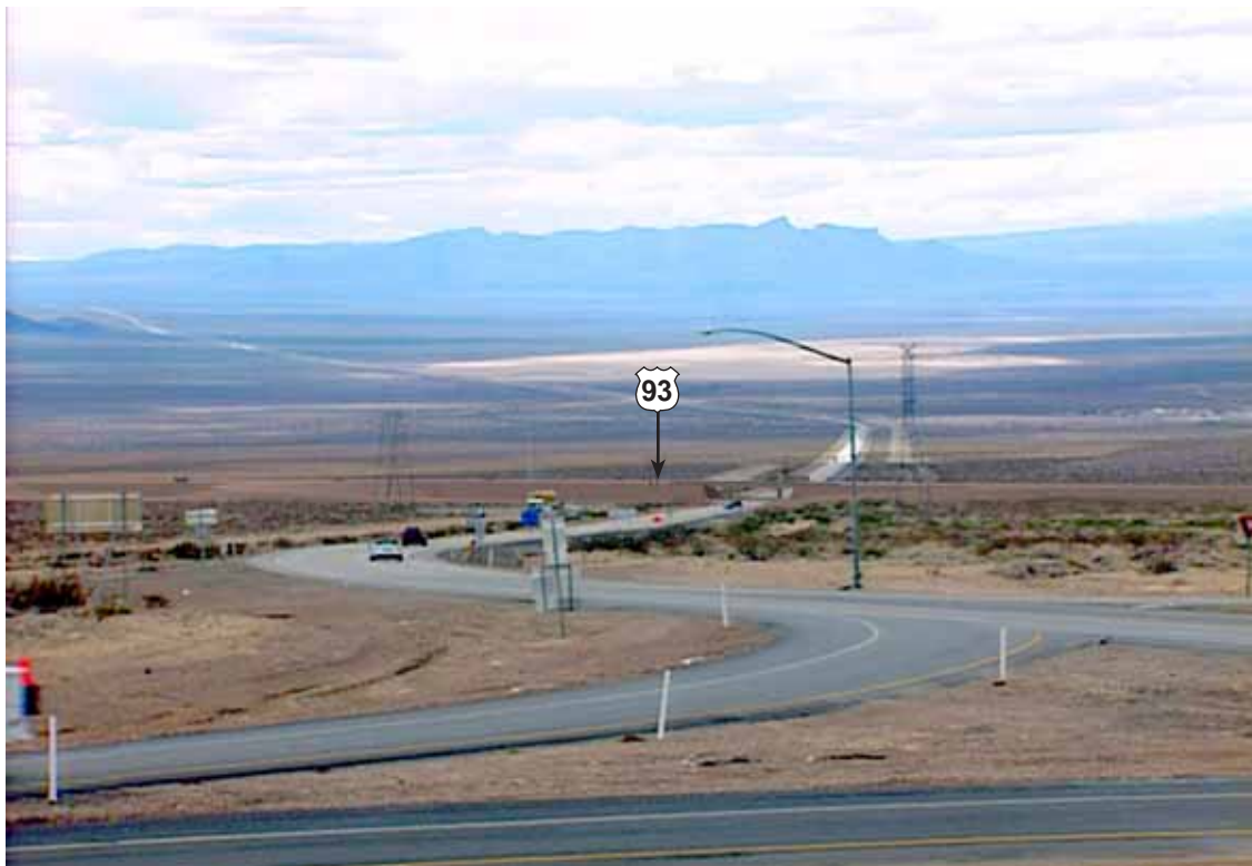
Simulated view looking south toward U.S. 95 near its intersection with U.S. 93. As shown, U.S. 93 would be an elevated crossing over U.S. 95.
