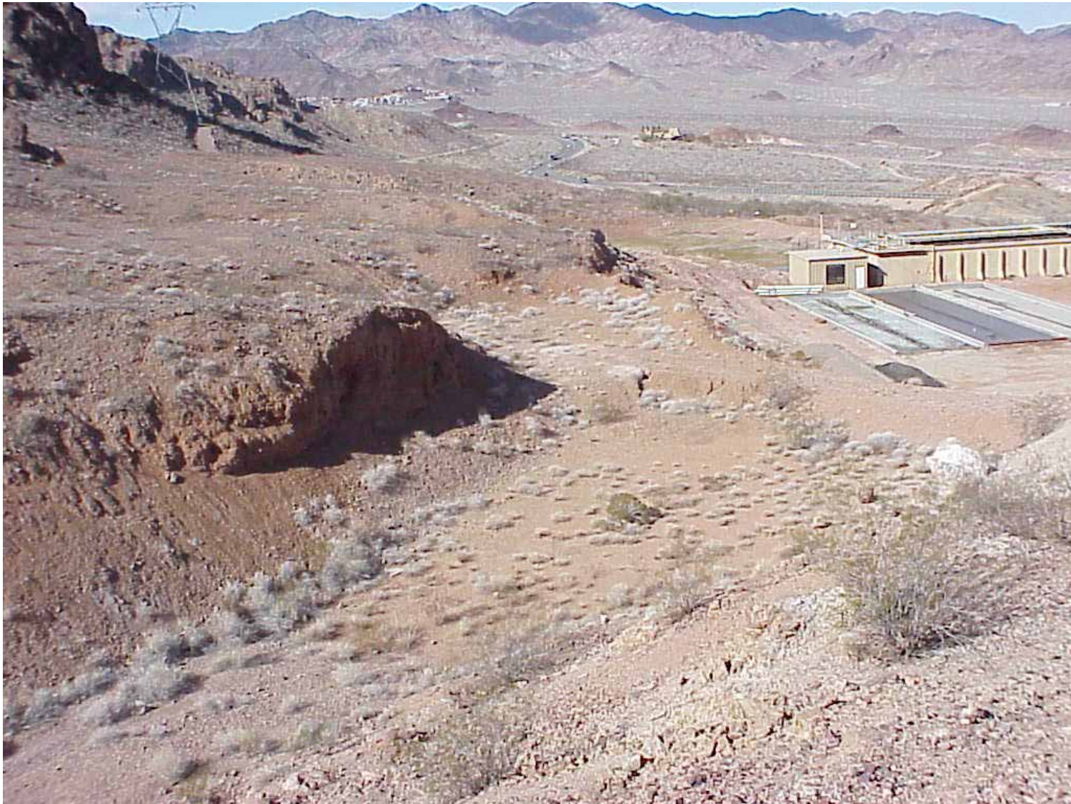
FIGURE 4-7 WASH CROSSING B-9 (CUTOFF AT WASTEWATER TREATMENT FACILITY) LOOKING NORTH - ALTERNATIVES B AND C BOULDER CITY/U.S. 93 CORRIDOR STUDY ENVIRONMENTAL IMPACT STATEMENT
