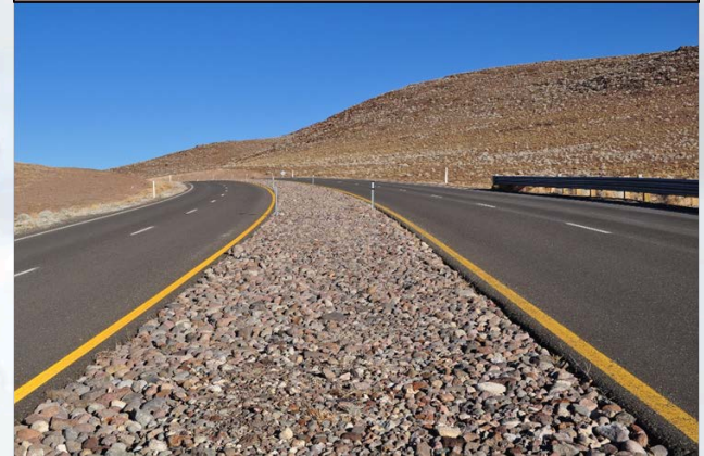
Removal and Replacement of Median Rock Mulch
