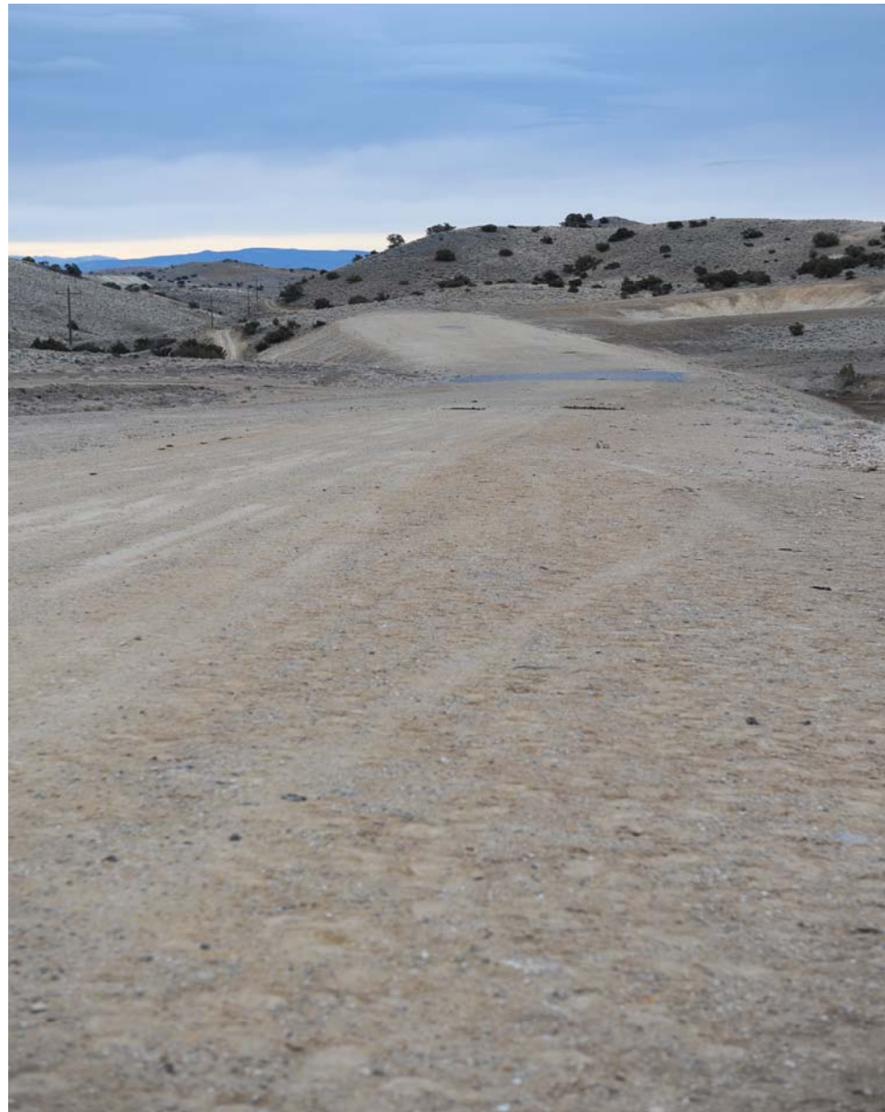
Photo #1: Station 470 – End of graded roadway
