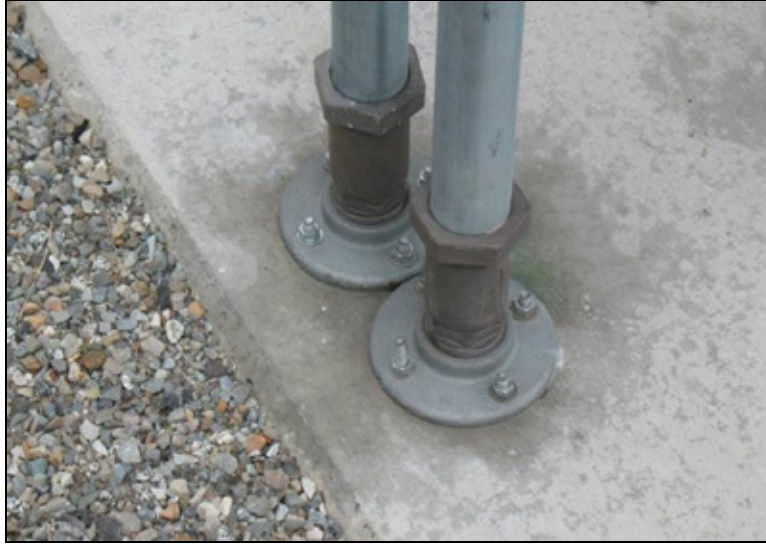
Figure 6-2. Two frangible connections
