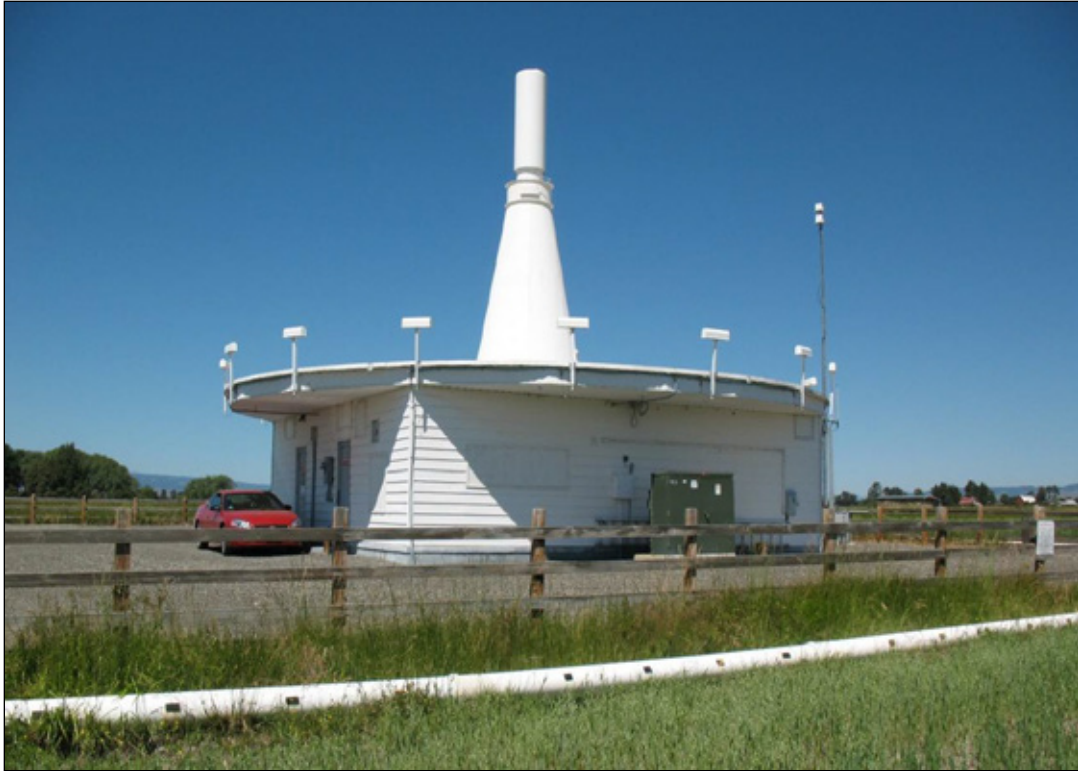
Figure 6-27. Enroute VHF Omnidirectional Range (VOR) facility
