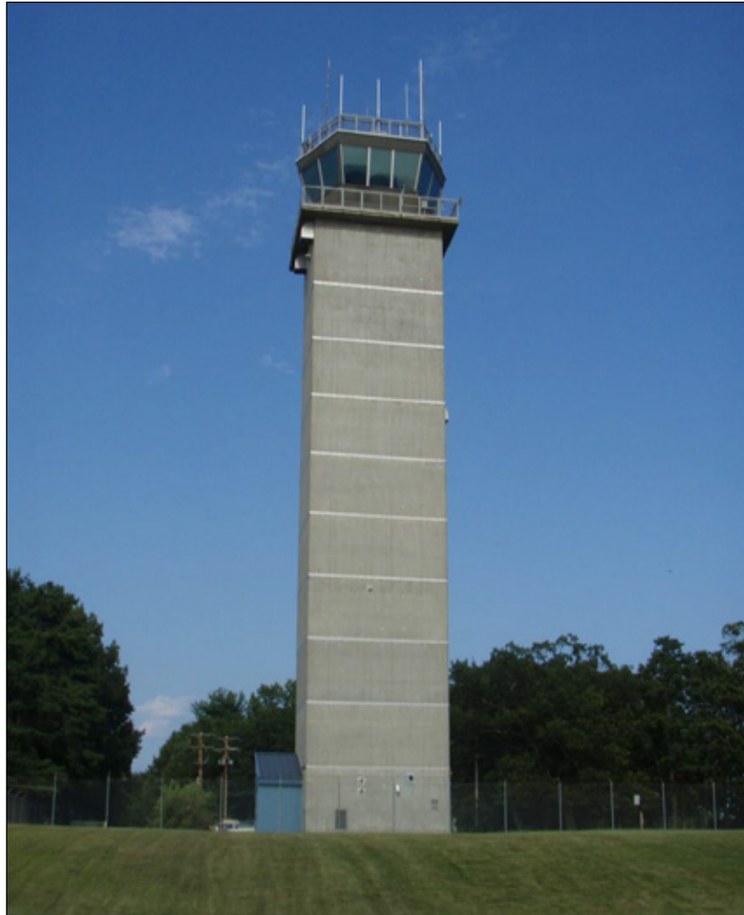
Figure 6-3. Airport Traffic Control Tower (ATCT) facility
