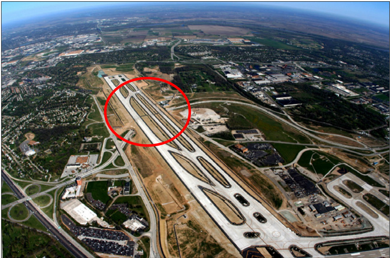
Figure 7-1. Tunnel under a runway and parallel taxiway
