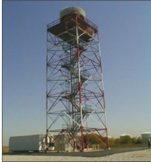
Figure 6-6. Precision Runway Monitor (PRM) facility
