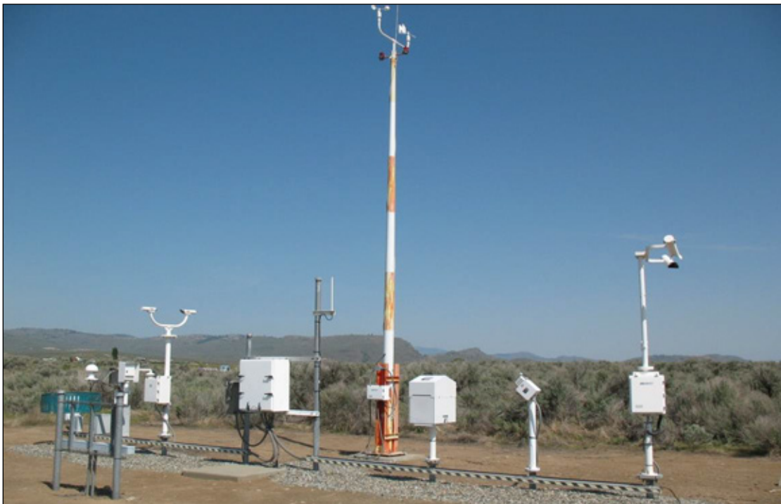
Figure 6-33. Automated Surface Observing System (ASOS) weather sensors suite
