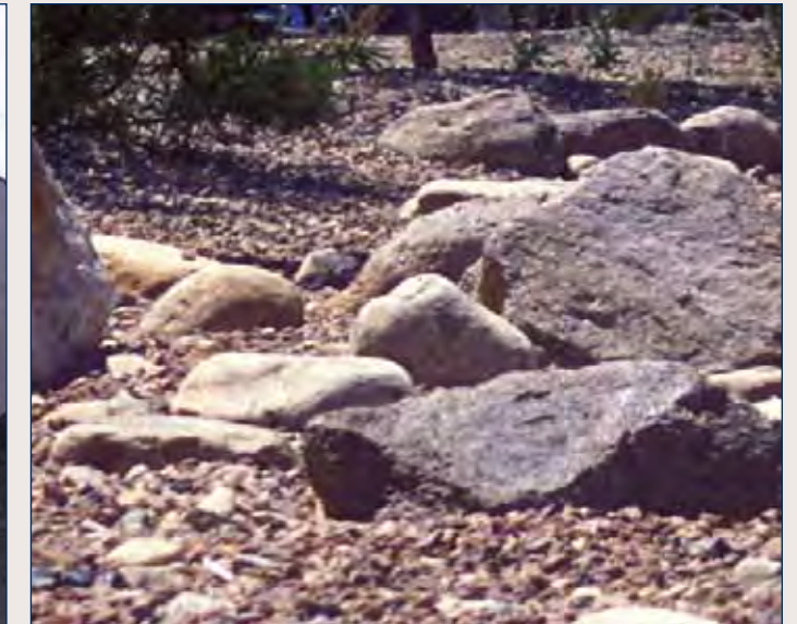
(3) Rock bed drainage allows water to infiltrate and provide water for adjacent plant materials.
