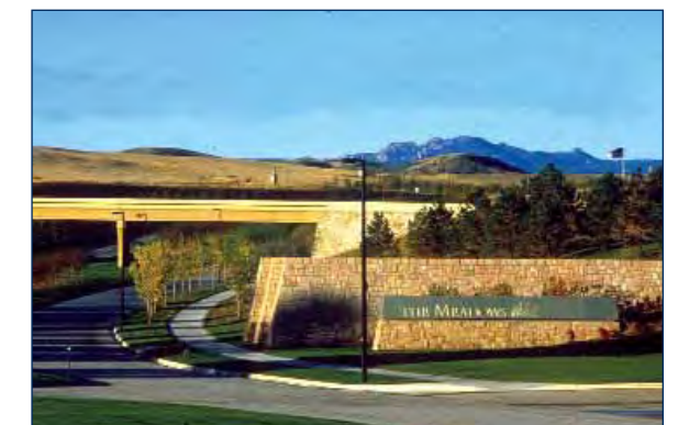
(5) Example of a community gateway incorporated into retaining wall and bridge structure.
