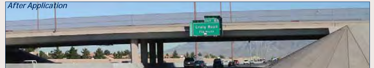
(1), (2) Appropriate coloring of bridge enhances visually quality
