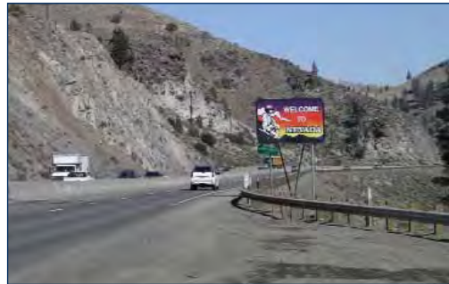
(1) This is the existing entry into Nevada from California along I-80.
