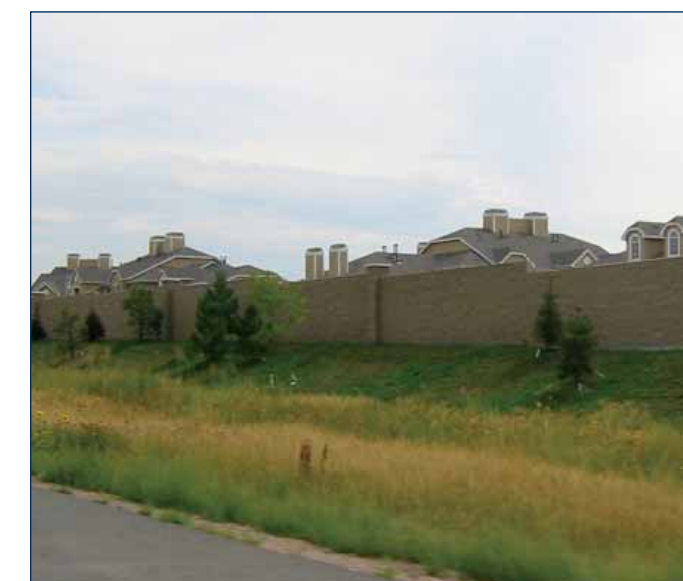
(12) Earth berms or embankment slopes are effective as sound barriers and should be used along or in combination with partially depressed road profiles. This can avoid walls where sound attenuation is required.
