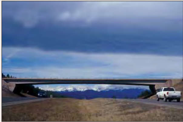
(1) This bridge on I-70 near the continental divide in Colorado was constructed without center piers to frame the view of the mountain range beyond. This underpass window enhances the view for the driver and creates a focus on high visual quality.
