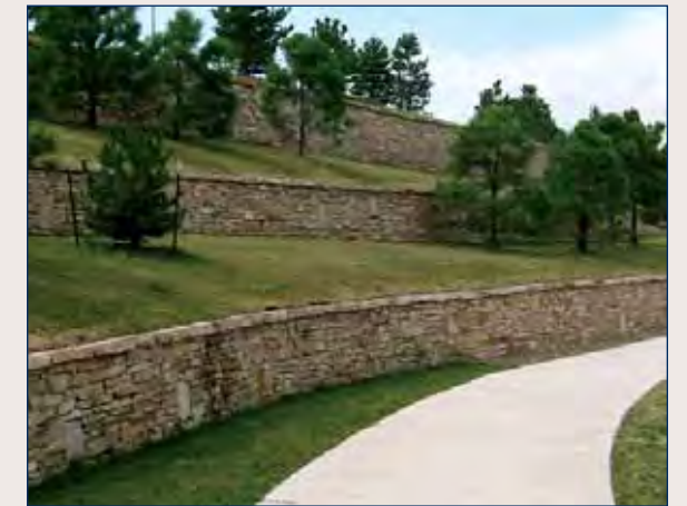
(6) Retaining walls provide space for pedestrian walkways.
