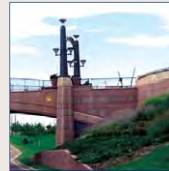
(3) Lights are incorporated in bridge design as a feature of the approach.
