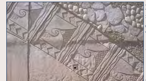
(5) Sound wall with decorative imprint motif created with custom form liner. This is both imprint as well as "additive relief" to project beyond the wall surface.
