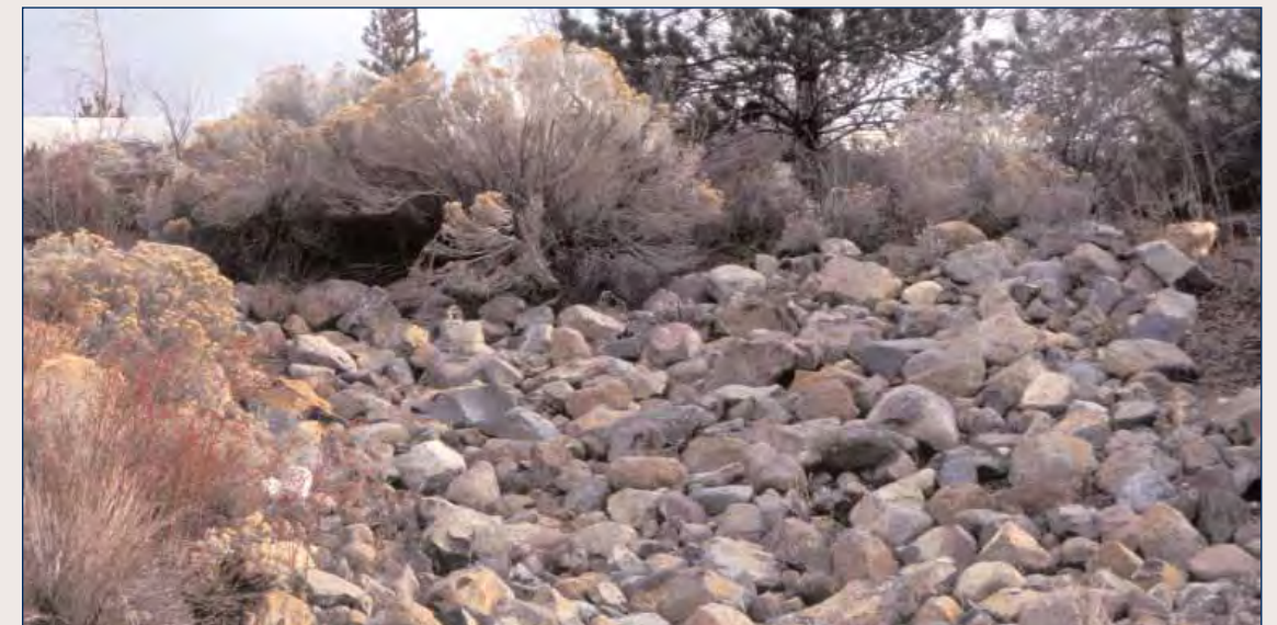
(2) Large-scale ground cover stone placement of various sizes may be utilized for slope stabilization.
