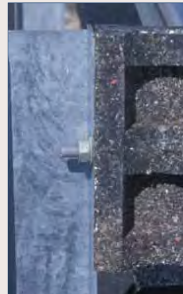
(3) Materials like this recycled plastic modular unit can be used in roadway construction.
