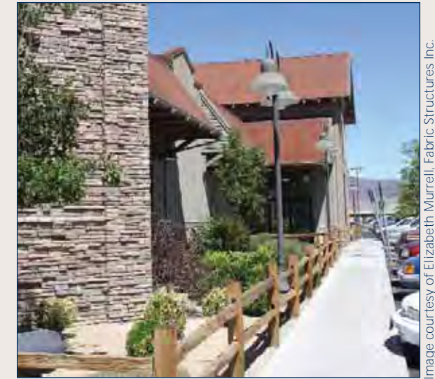
(2) The National Park architecture found in the Sierra Nevadas is reflected in materials.
