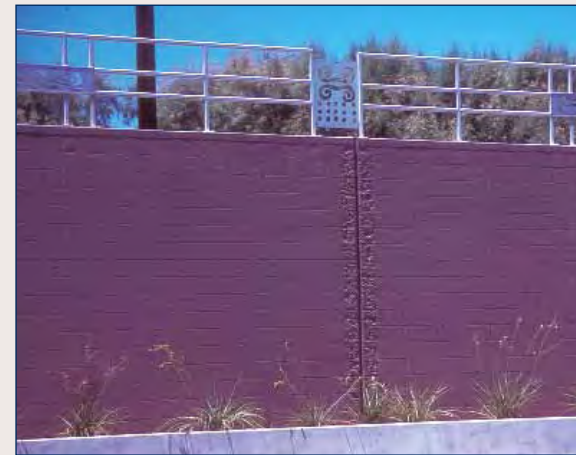
(5) Simple retaining wall patterning, railing design, and landscape palette. The wall is separated from the concrete barrier with the space and planting area.
