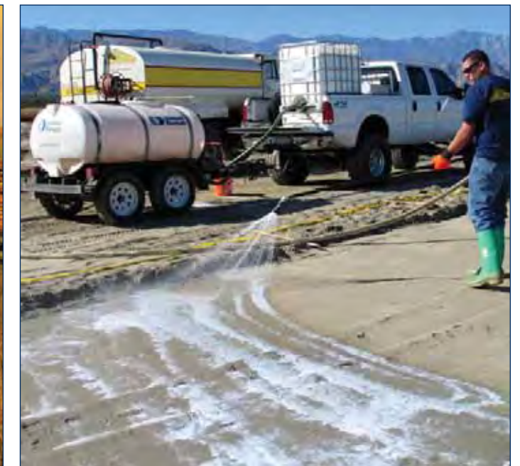
(5) Application of soil stabilizer aids in dust and erosion control.
