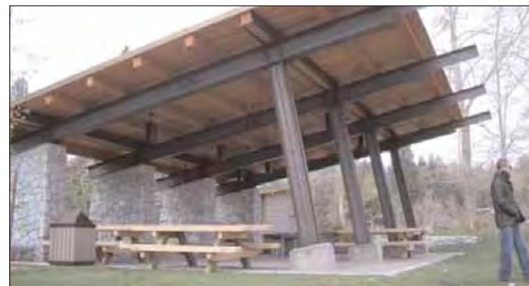
(2) Shade structures at interpretive rest area with table, benches, and shade structure that frames significant views.
