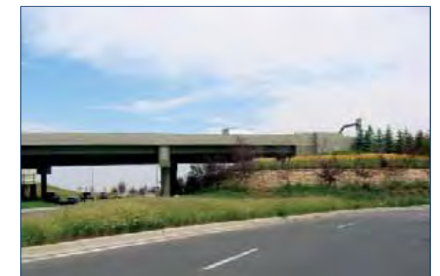
(4) Community gateway incorporated into retaining wall and bridge structure are appropriate for town entries along the rural study area.
