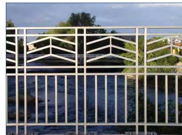
(4) Custom pedestrian bridge rail highlights a crossing point.
