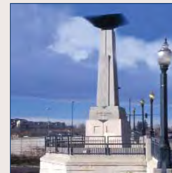
(5) This is an example of a monumental light incorporated into road design.
