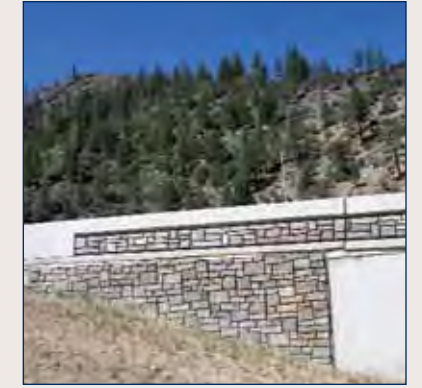
(5) Bridge features reflect local stone materials.
