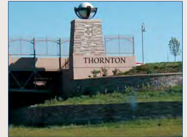
(3) Bridge design integrated into retaining wall with landscape planting creates gentle slopes and area for landscape planting.
