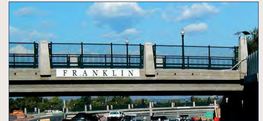
(7) Emboss names on the bridge span to provide wayfinding for the motorist in the urban Reno/Sparks area.
