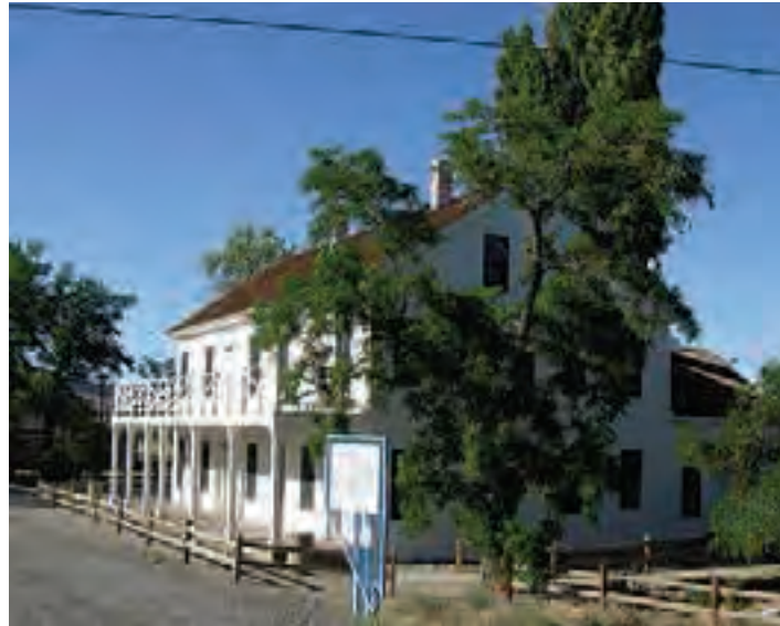
(3) Historic buildings provide opportunities for rest areas and interpretive features.
