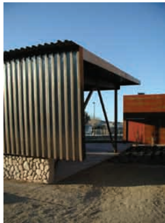
(7) Shade structures add architectural and cultural interest to rest areas.
