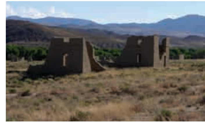
(2) Interpretive elements should be provided for important historical elements such as the ruins of Fort Churchill.
