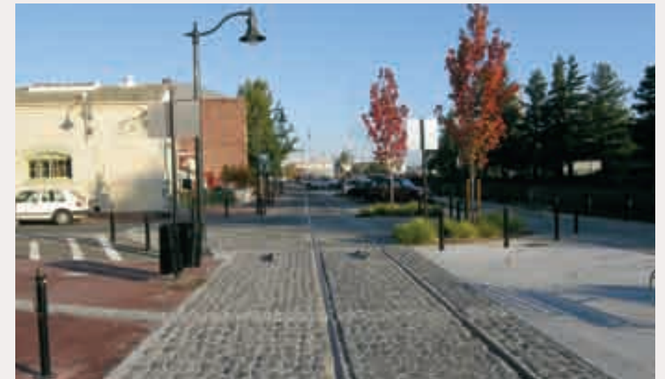
(5) Choice of paving reflects local character. In the example above, railroad tracks have been converted to a pedestrian promenade that recalls an aspect of the town's history.
