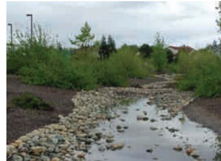
(2) Water harvesting features can be combined with regionally adapted plantings where seasonal runoff is common.
