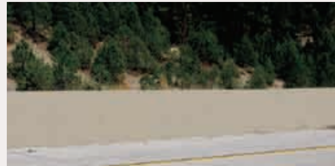
(1) Stained concrete barriers should use colors from the design segment’s color palette.
