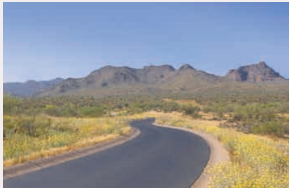
(1) The enhanced native softscape type is used in transition zones from rural open highways to developing communities.
