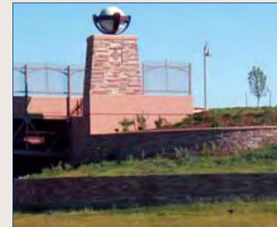
(3) Bridge design integrated into retaining wall with landscape planting to create moderately steep slopes and terraces for planting.
