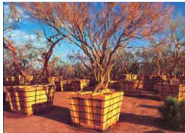
(2) Appropriate tree boxing techniques are necessary for proper transfer of tree materials during construction.
