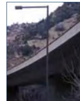
**(5)** This is an example of a colored shoebox style fixture on a steel pole.
