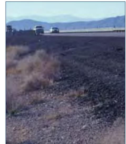
**(4)** Existing condition of asphalt millings being placed along the shoulder should be reused in repaving projects.
