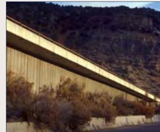
(2) An example of a cantilevered retaining wall with a simple, consistent use of materials. Vertical joints are most compatible with the finish.
