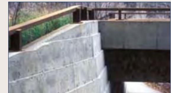
(9) Pedestrian underpass integrated into highway bridge design, rather than separate structure design. Height of opening allows light into underpass.
