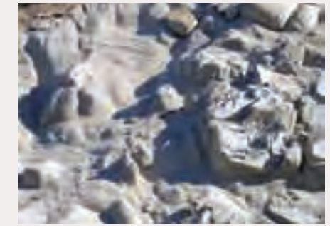
(3) Avoid securing slopes with concrete facing when possible. When necessary, use colored concrete that resembles natural rock face textures.
