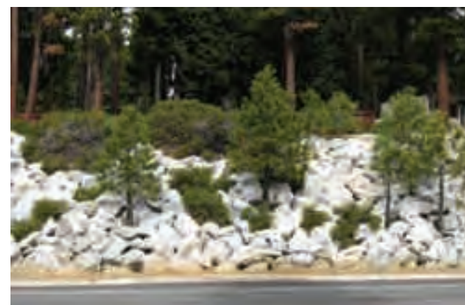
(1) Native rock and vegetation add aesthetic value while stabilizing slopes.
