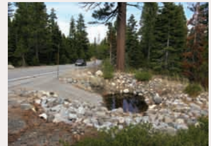
(4) Small detention features lined with rock and native vegetation allow slow infiltration of runoff.
