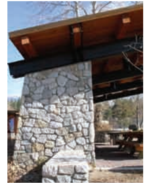
(2) The design of rest area structures should incorporate plantings, materials, and landscape features that reinforce the corridor’s design theme.
