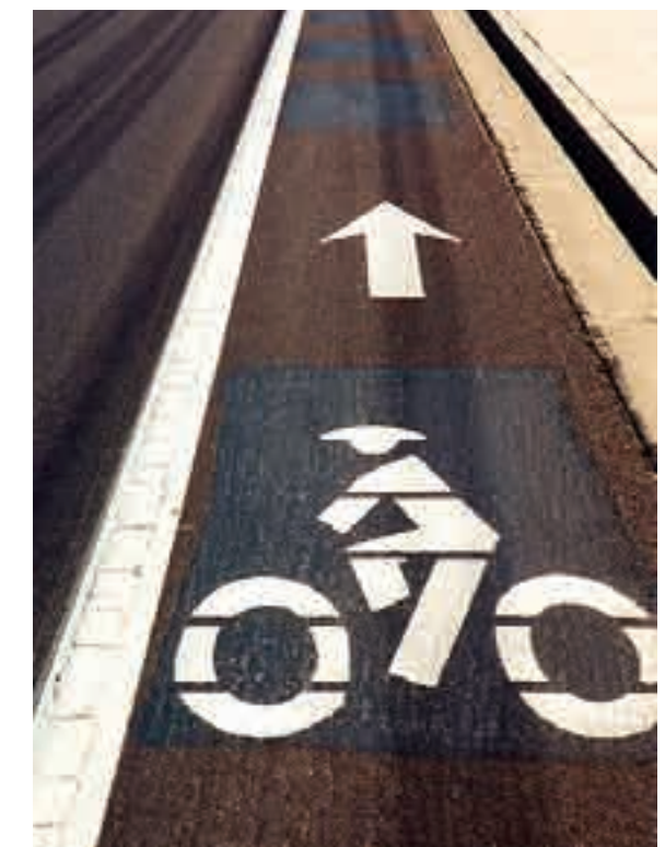
(4) Bike lanes should be signed, striped, and designated with a bike symbol.
