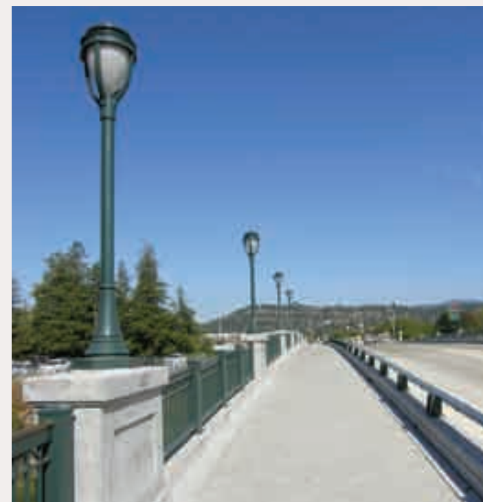
(13) Architectural details and columns provide opportunities accentuate prominent drainages.
