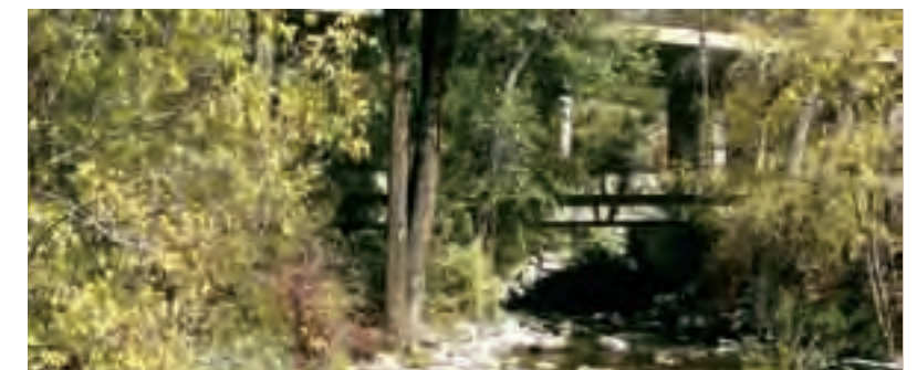
(9) Roadway design considers wildlife movement through drainages. Fill of canyons is minimized.
