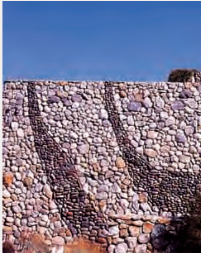
(1) The Corridor Plan guides the development of project specific design through established design objectives and design guidelines.
