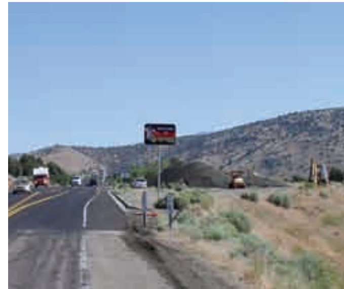
(2) The existing entry into Nevada near Topaz Lake lacks a visually inviting aesthetic.
