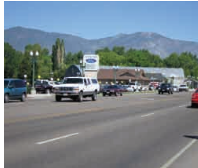
(2) The wide appearance of the existing roadway encourages faster travel speeds and discourages pedestrian movement.
