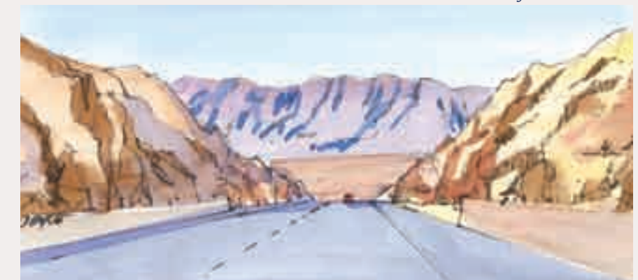
(5) Preferred re-sculpted rock cut changes artificial slope banks into naturally occurring landforms. Plan cuts that terrace, bench, and use bedding planes found in rock formations are the final design of any rock slope.
