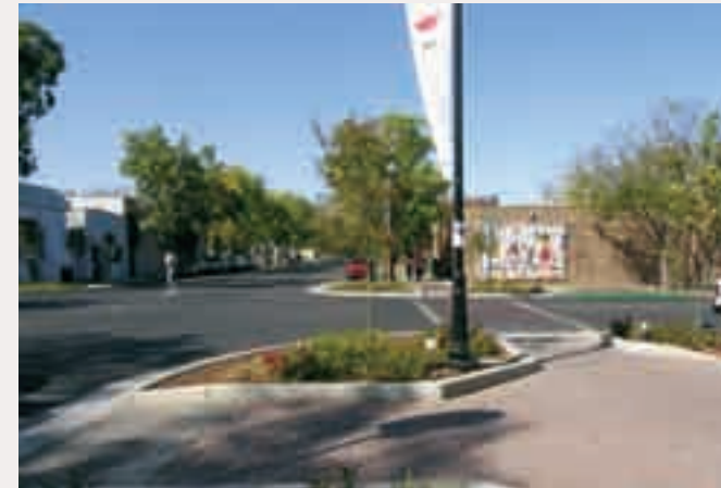
(6) Tighter turning radii provide sidewalk space for landscape enhancements and clear delineation of crossing points.
