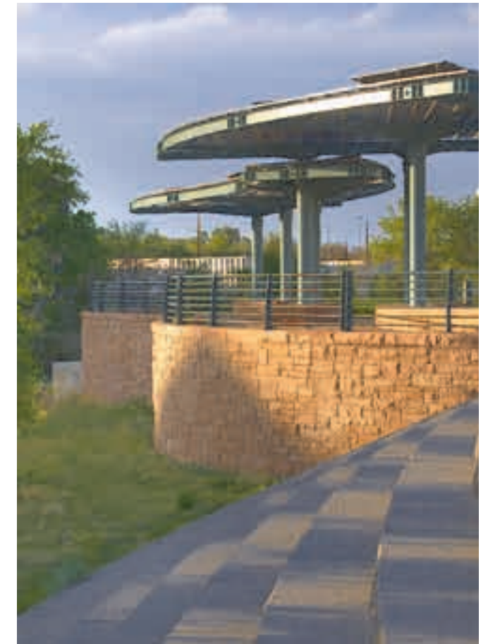
(5) A sheltered structure at a point of interest gives travelers a protected place to enjoy views.
