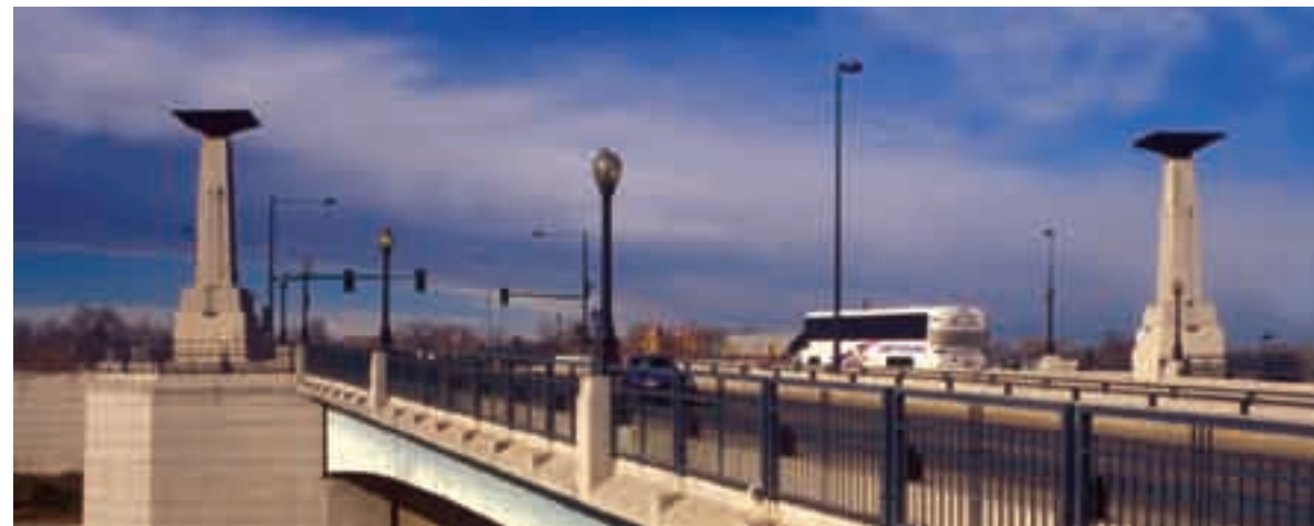
(8) Structures within the Edge of the Sierra Crossroads should utilize colors and materials representative of the surrounding landscape. The Plumb Lane interchange establishes the gateway into the Reno/Tahoe area from the international airport, justifying landmark treatments.
