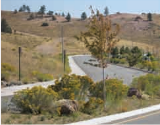
(2) Low-water use plant species selected for landscape improvements along roadways help to conserve water. Native vegetation patterns should be used as a reference for landscape design.
