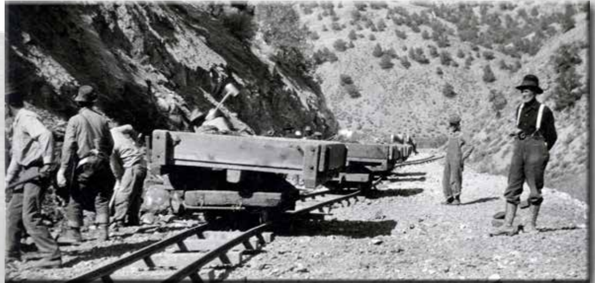
Building mountain roads, such as this one over the Carroll Summit proved to be treacherous and slow work
