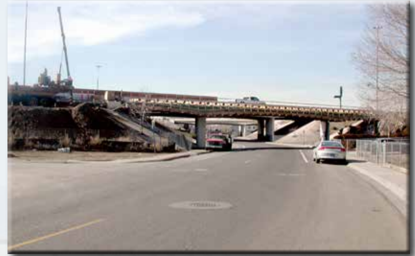
Interstate 80/U.S. Highway 395 construction in Reno, 2004
