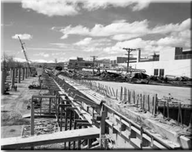
Construction on I-80 in Sparks, 1966
