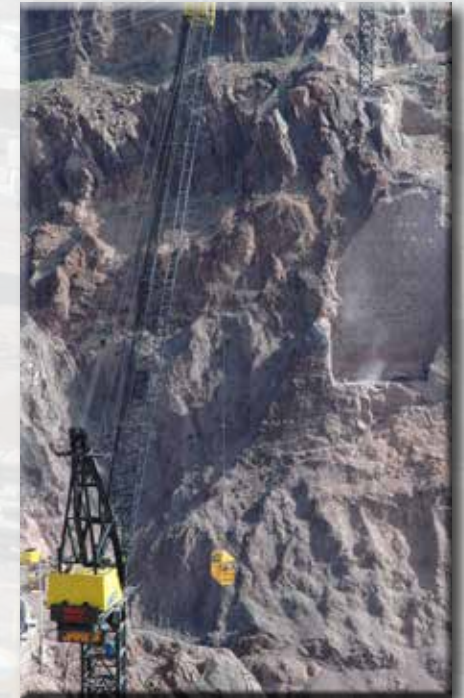
Hoover Dam bridge work, 2006
