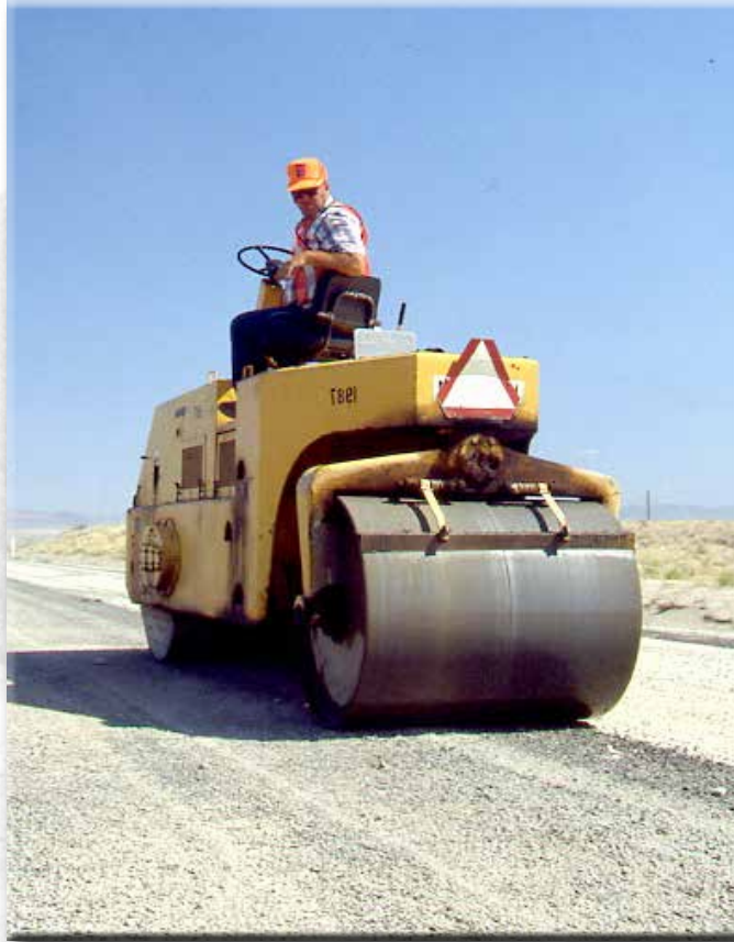
Paving U.S. Highway 50 in 1988
