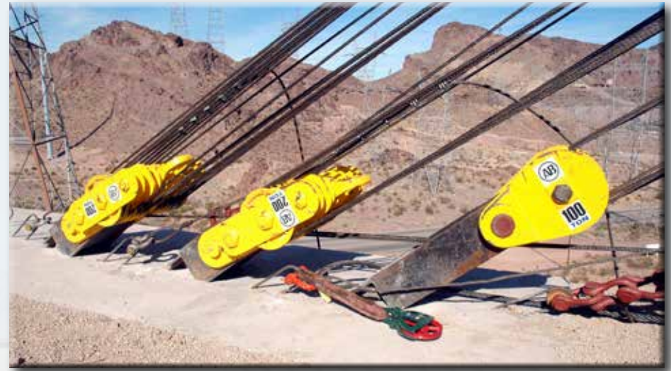
Hoover Dam bridge work, 2006
