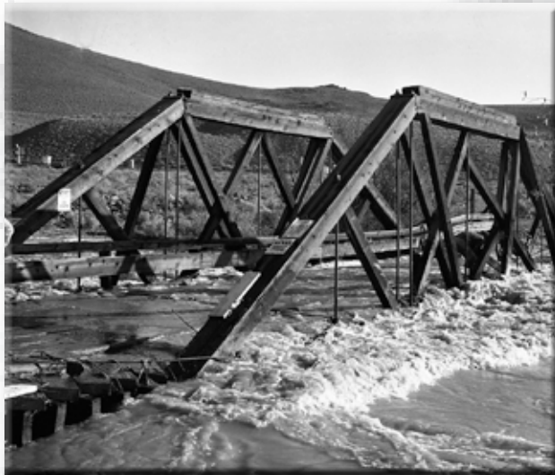
A bridge is nearly wiped out by flood waters
