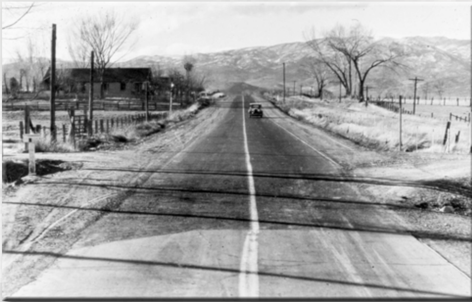
NDOT crews initially used solid white lines for the centerline of roadways, but the cost and availability of paint became challenging, prompting the department to convert to dotted center lines
