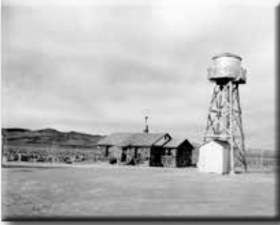
A rural highway maintenance station
