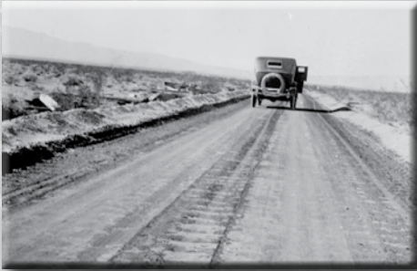
Completed oil-sand surface
