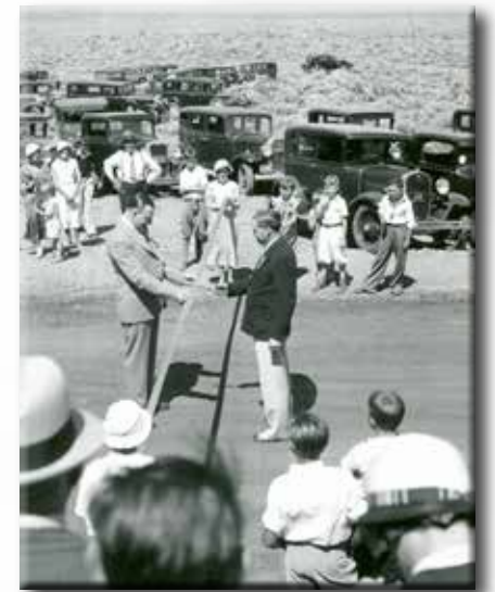
Groundbreaking events to introduce the public to new roads, and show how taxpayer money was used, have been commonplace with NDOT for decades
