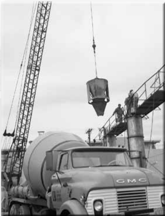
Road construction equipment in action, 1966
