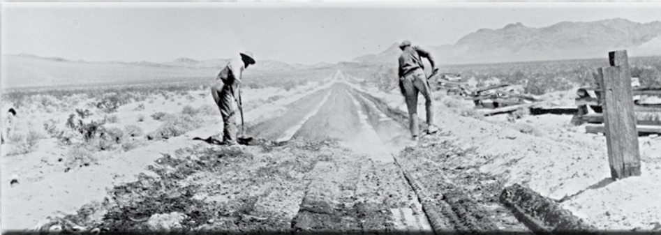
Highway workers applying sand
