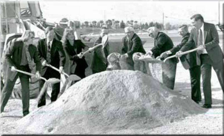
Rancho Road reconstruction groundbreaking, 1996
