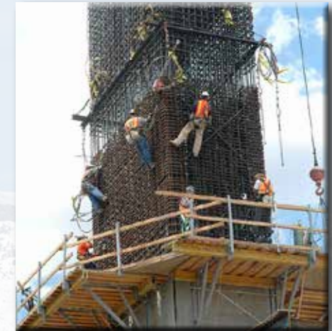
Galena Creek bridge work
