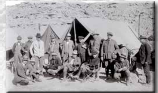
Highway department survey crew
