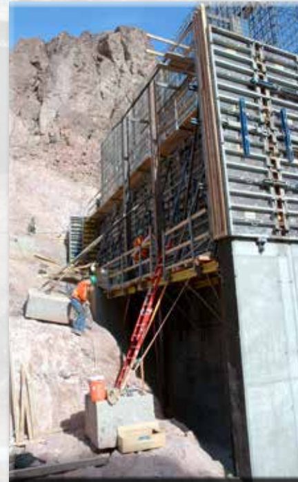
Hoover Dam bridge work, 2006
