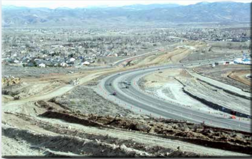
Carson City Freeway construction, 2004
