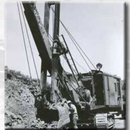
Crews work on the Geiger Grade, which was a critical route that linked Virginia City and Lake Tahoe
