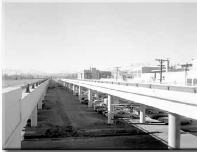
Construction finished on I-80 in Sparks, 1966
