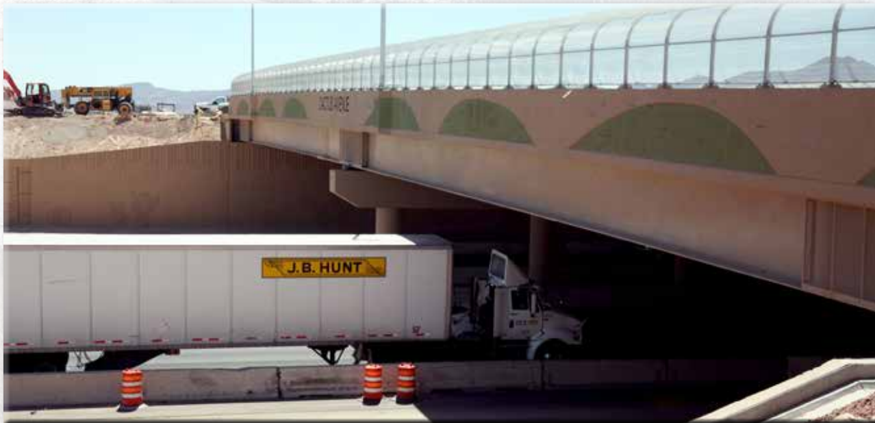
The Cactus Avenue overpass across Interstate 15 was completed in 2014, providing an important east-west arterial for residents in the southern portion of Clark County
