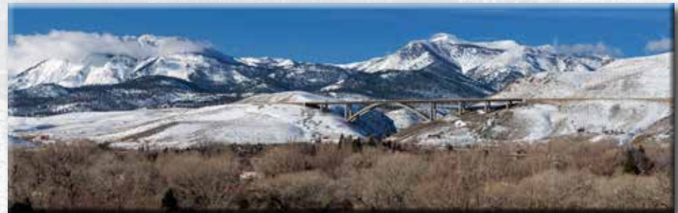
Completed Galena Creek Bridge
