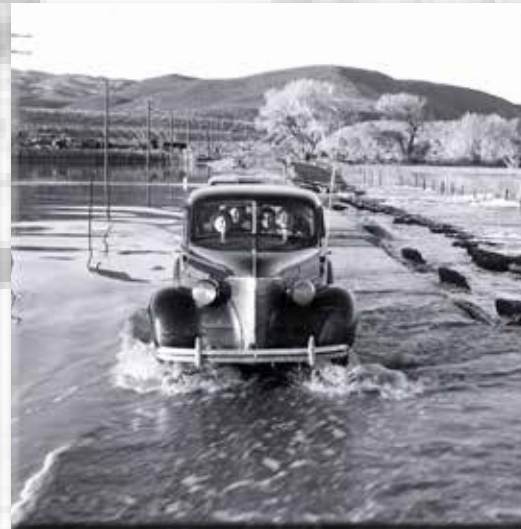
A motorists traverses a flooded road near Reno
