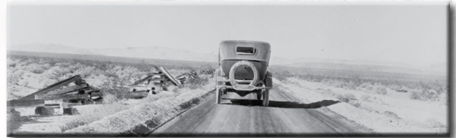
Freshly-sanded roads did away with much of the ruts providing much smoother roads in the 1920s
