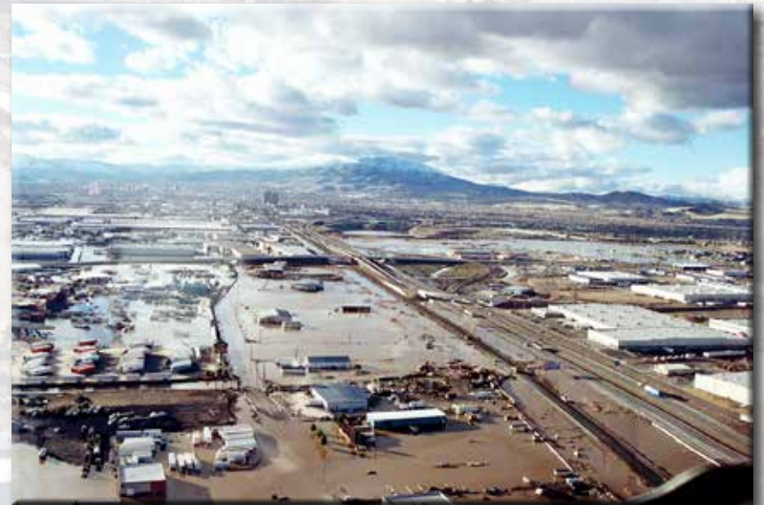
NDOT personnel was busy in 1997 when flooding ravaged Reno and Sparks
