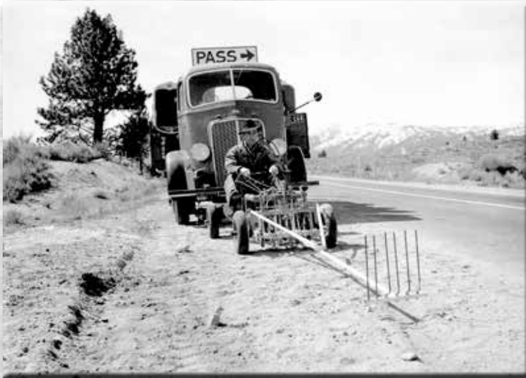
Striping the road
