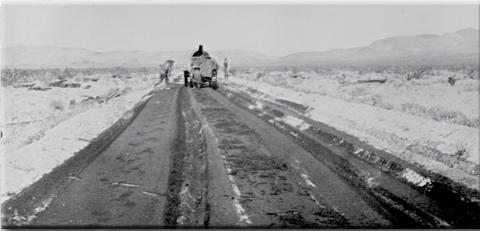
Applying oil to new roads offered a far more smooth surface for travelers
