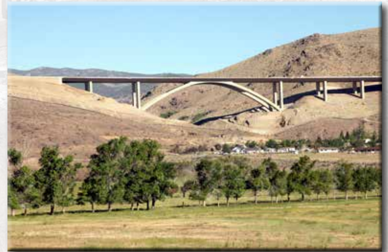
The Galena Creek Bridge along Interstate 580
