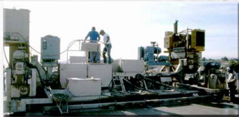
Crews work on Interstate 15 in 1985
