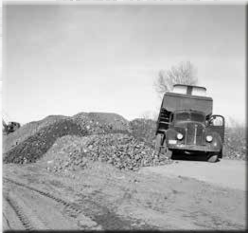
Clearing roads of debris after flooding has always been a priority for NDOT
