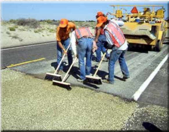
Paving takes place on U.S. Highway 50 in 1988
