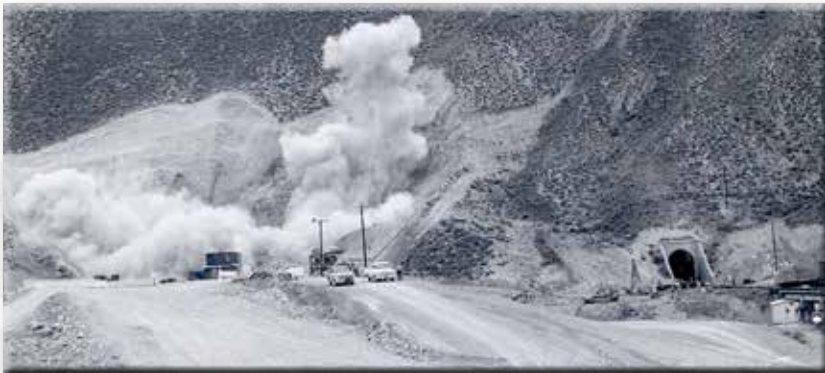
Blasting at Carlin Tunnels
