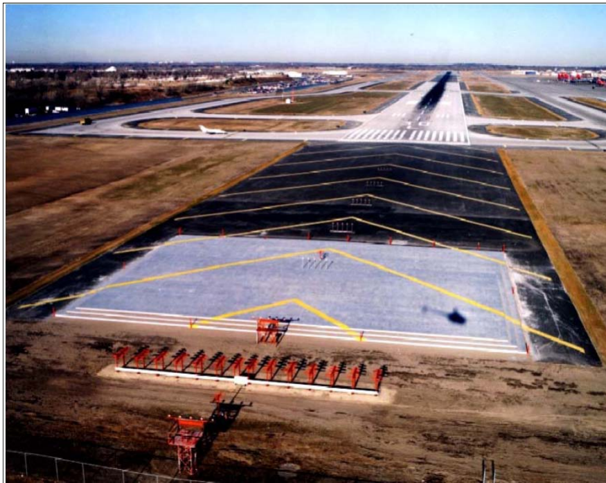
FIG 2-3-42 Engineered Materials Arresting System (EMAS)
