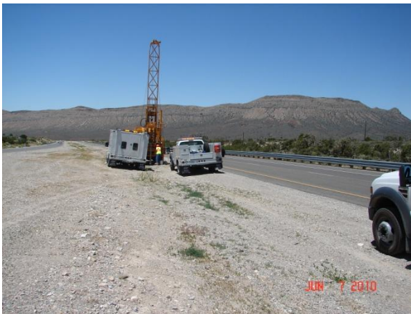
Drilling at CBP2.
