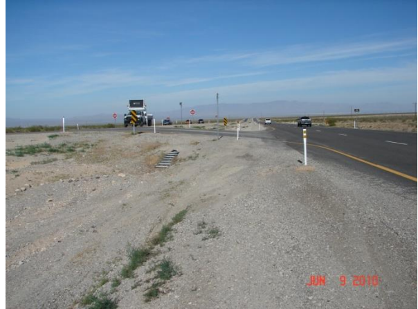
At station "X2" 1379+52 at CBP6 looking west.
