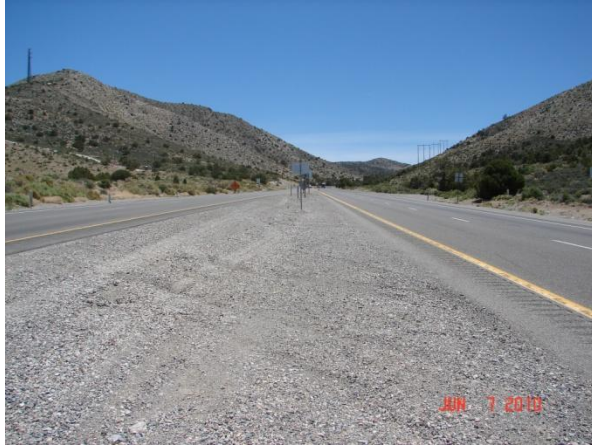
Beginning of project at station "X2" 1140+67 looking east towards Mountain Springs.
