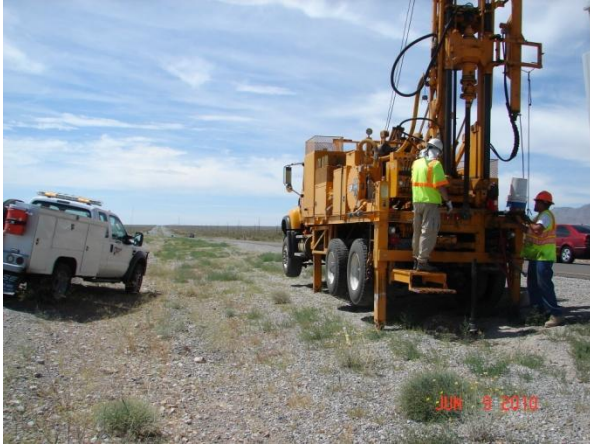
Drilling at CBP10.
