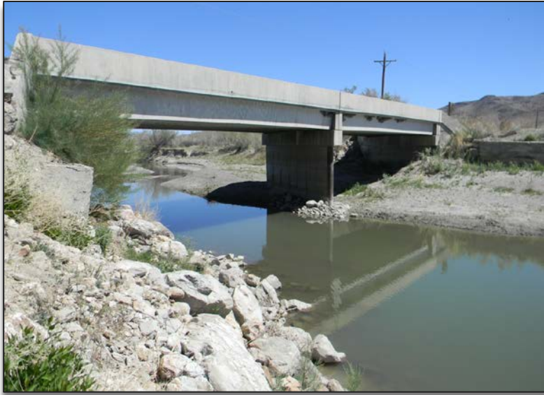
Eden Valley Bridge B-1658
