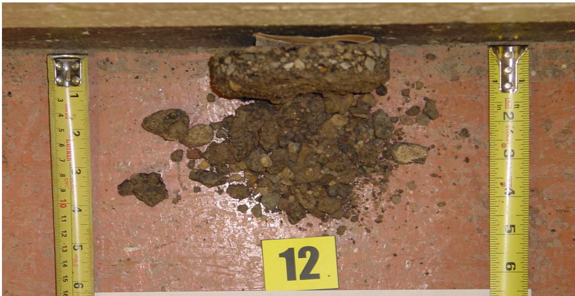
3 Years after Construction: Stripped and Fell Apart Pavement Condition: Good Condition
