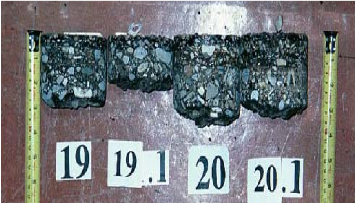
Before Construction: Light Stripping Pavement Condition: Transverse and Fatigue Cracking
