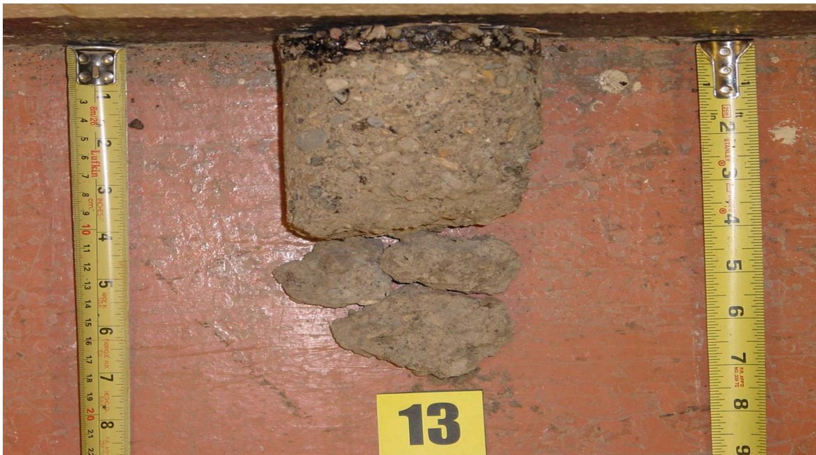
3 Years after Construction: Broke and Fell Apart Pavement Condition: Good Condition
