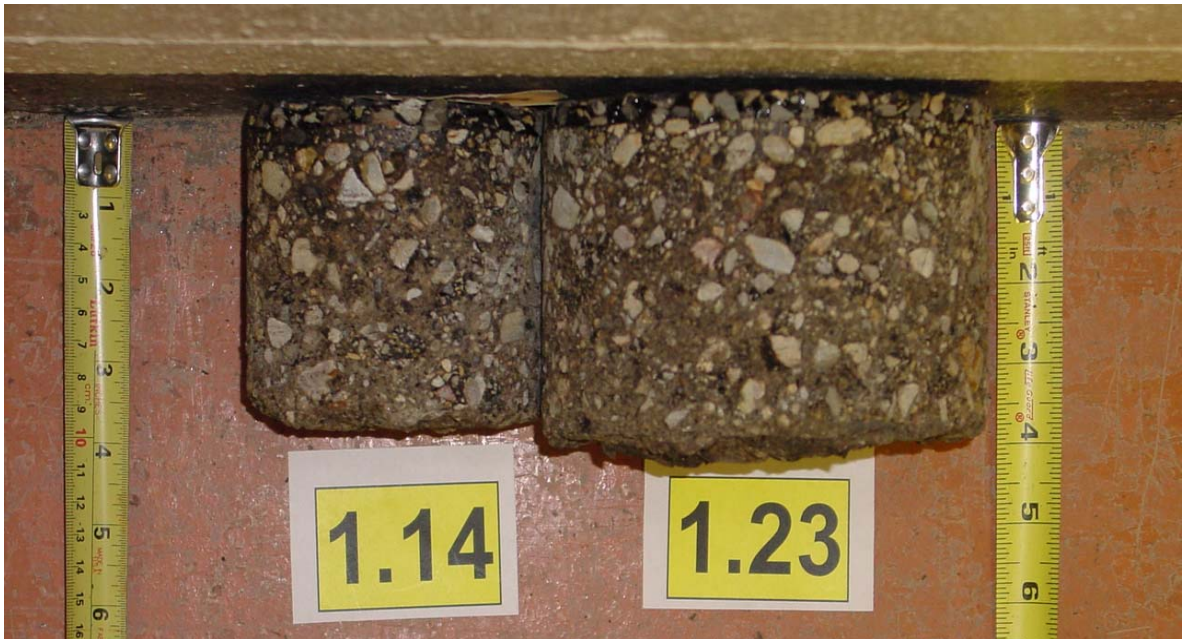
1 Year after Construction: Light Stripping Pavement Condition: Good Condition
