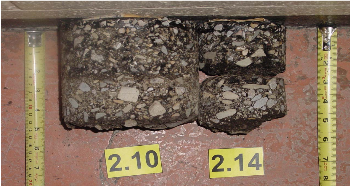
(a) 4 Months after Construction: Light to Medium Stripping and Delaminated Pavement Condition: Good Condition
