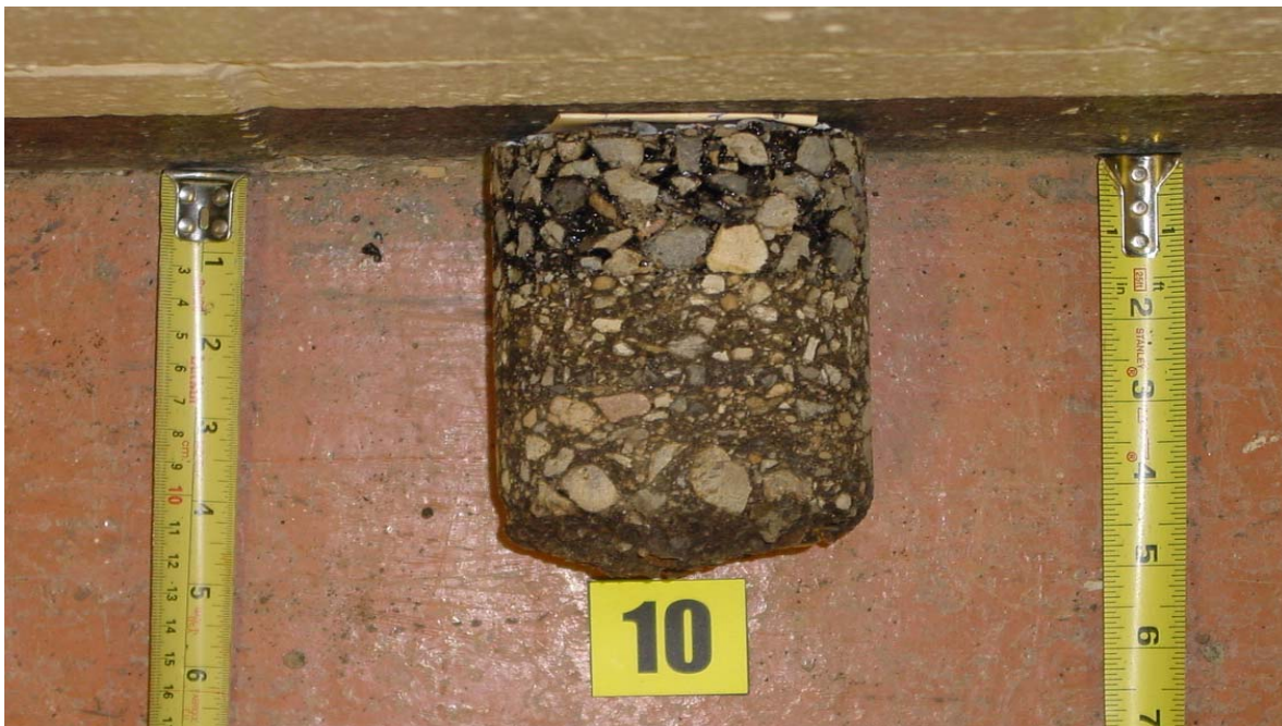
3 Years after Construction: Light to Medium Stripping Pavement Condition: Good Condition
