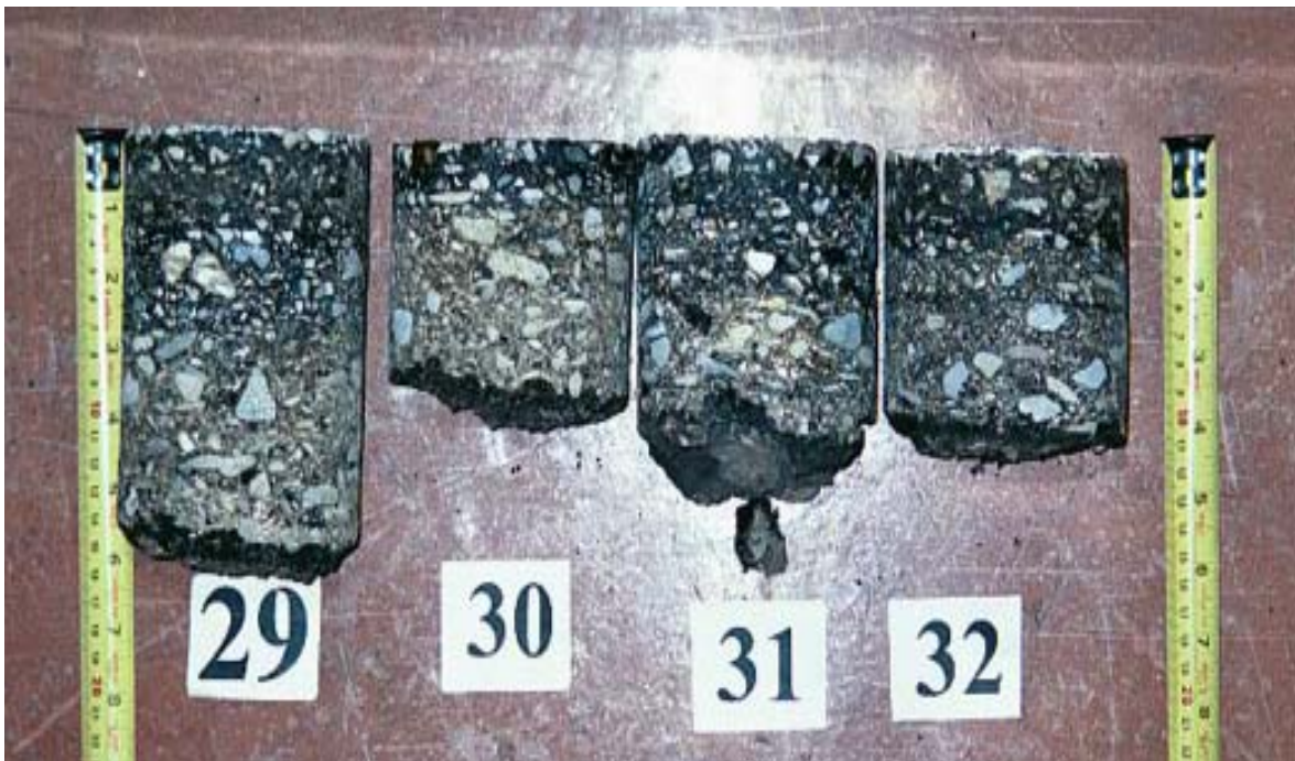
Before Construction: Light Stripping Pavement Condition: Transverse Cracking
