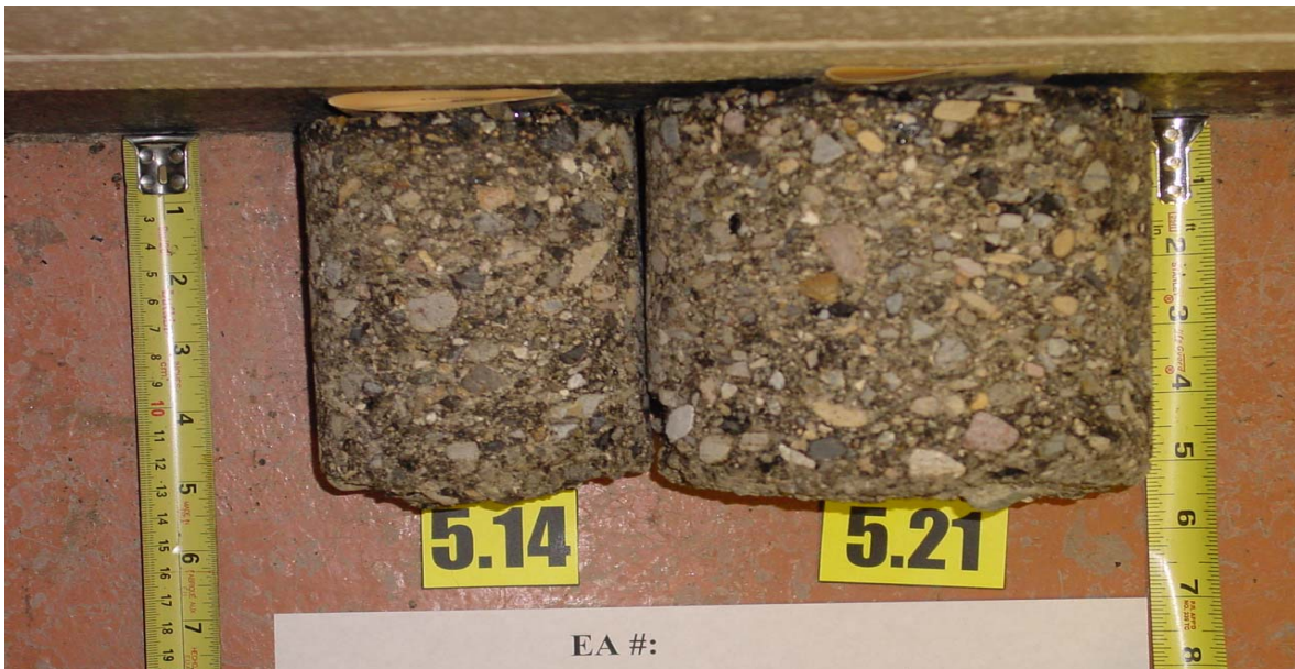
3 Years after Construction: Light Stripping Pavement Condition: Low Severity Transverse Cracking
