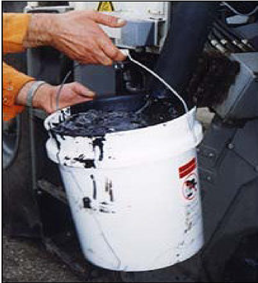
FIGURE 2.6a Foamed asphalt expands 15 to 20 times the volume of materials used separately (2).
