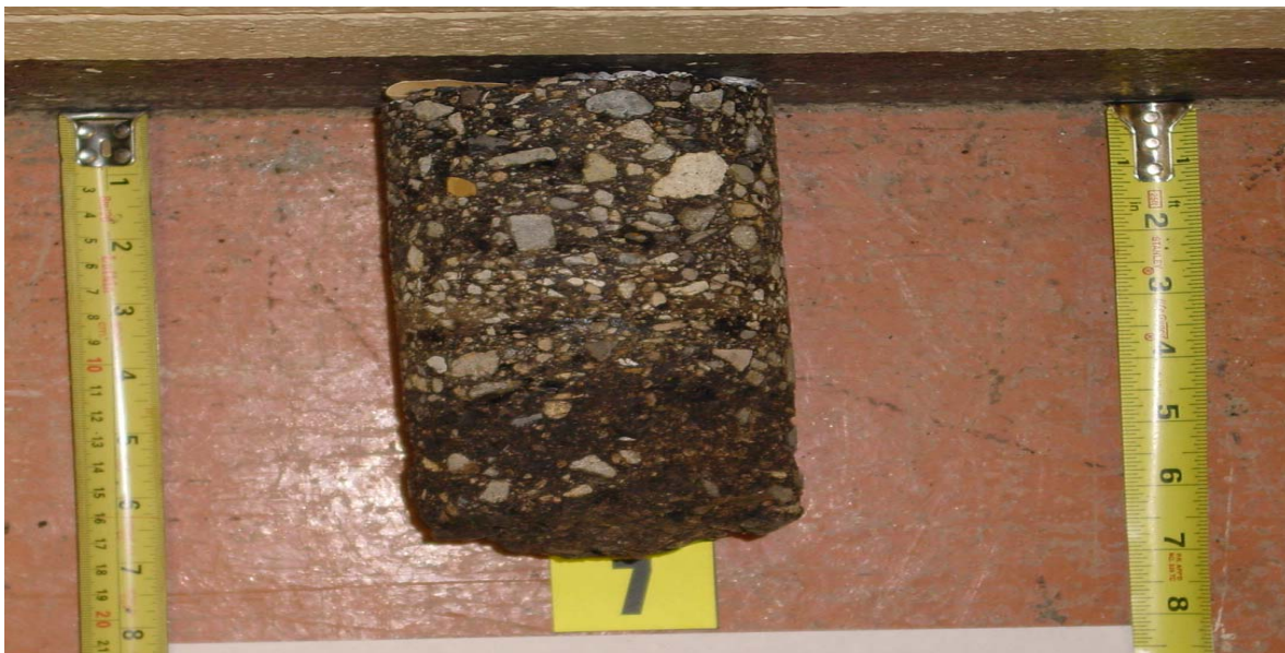
3 Years after Construction: Light to Medium Stripping Pavement Condition: Good Condition
