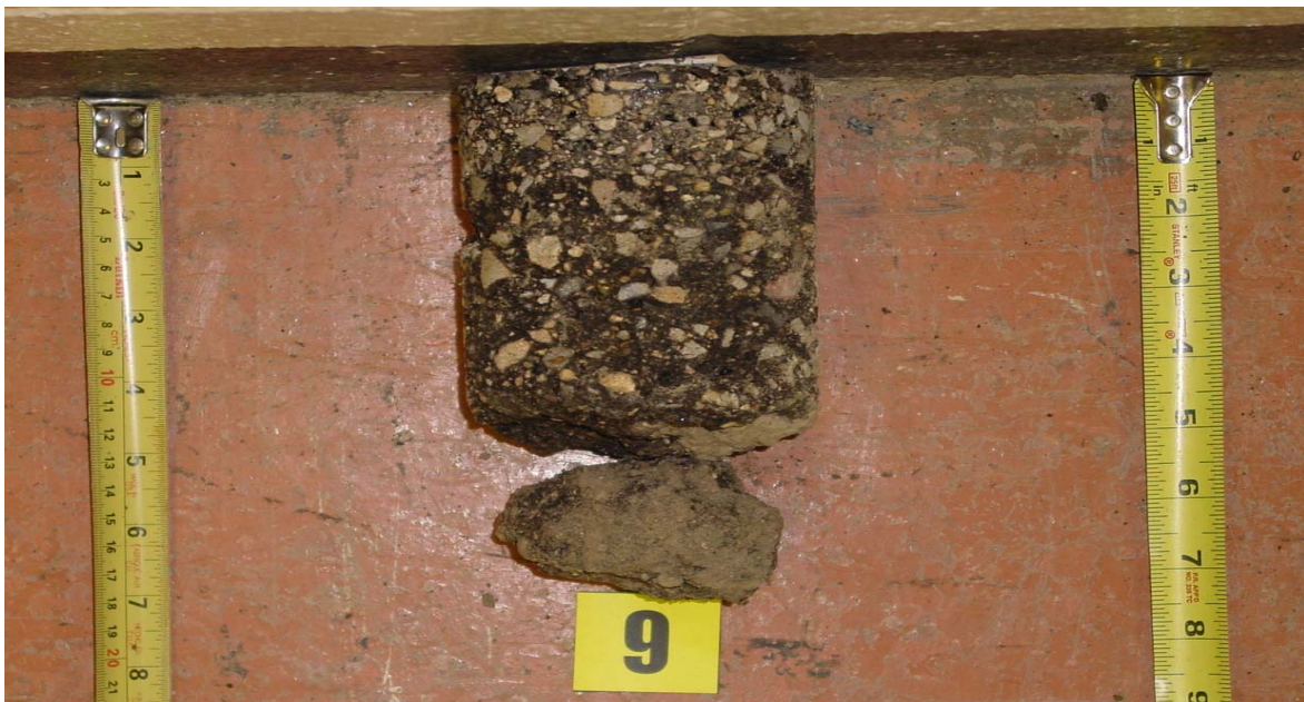
3 Years after Construction: Stripped and Fell Apart Pavement Condition: Good Condition
