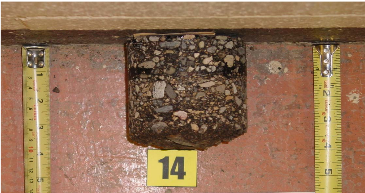
3 Years after Construction: Light to Medium Stripping Pavement Condition: Good Condition
