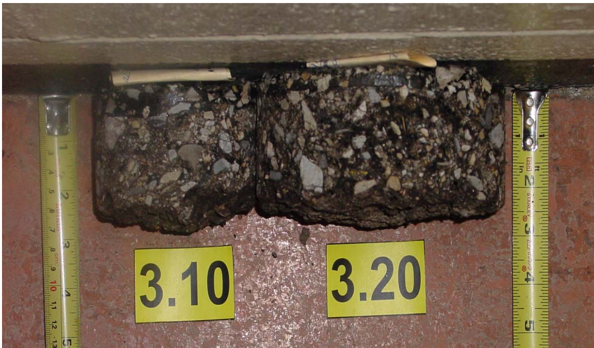
(b) 4 Months after Construction: Light Stripping Pavement Condition: Good Condition
