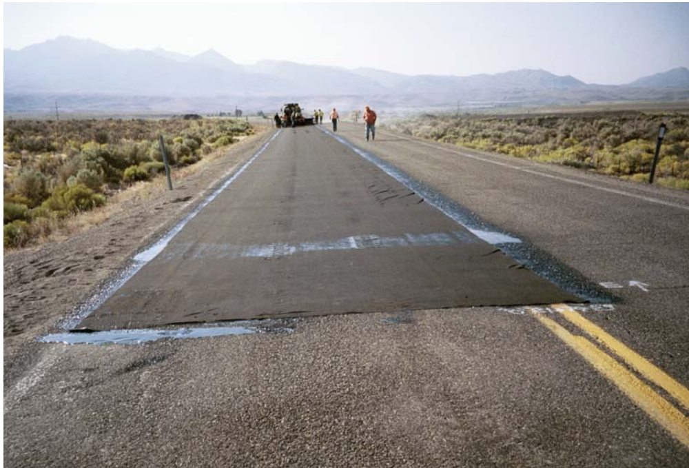
FIGURE 5.1a Nonwoven polypropylene geotextile fabric seated in tack coat.
