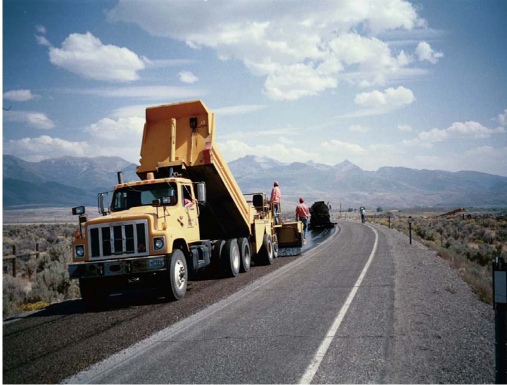
FIGURE 5.1b Maintenance personnel place chip seal.
