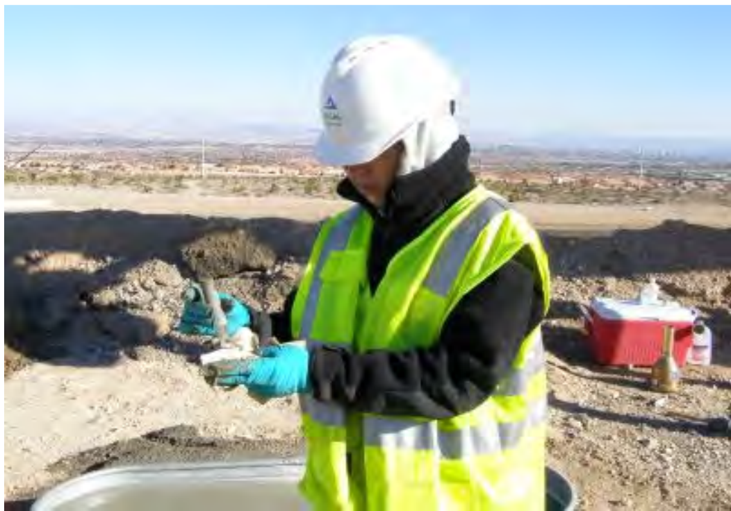
Figure 6.11: Sample collection for air void analysis test
