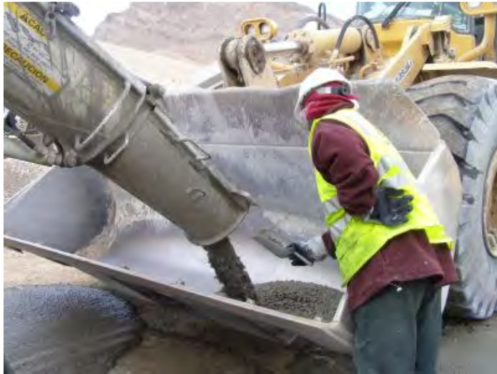
Figure 6.6: Visual inspection of fresh concrete before pumping
