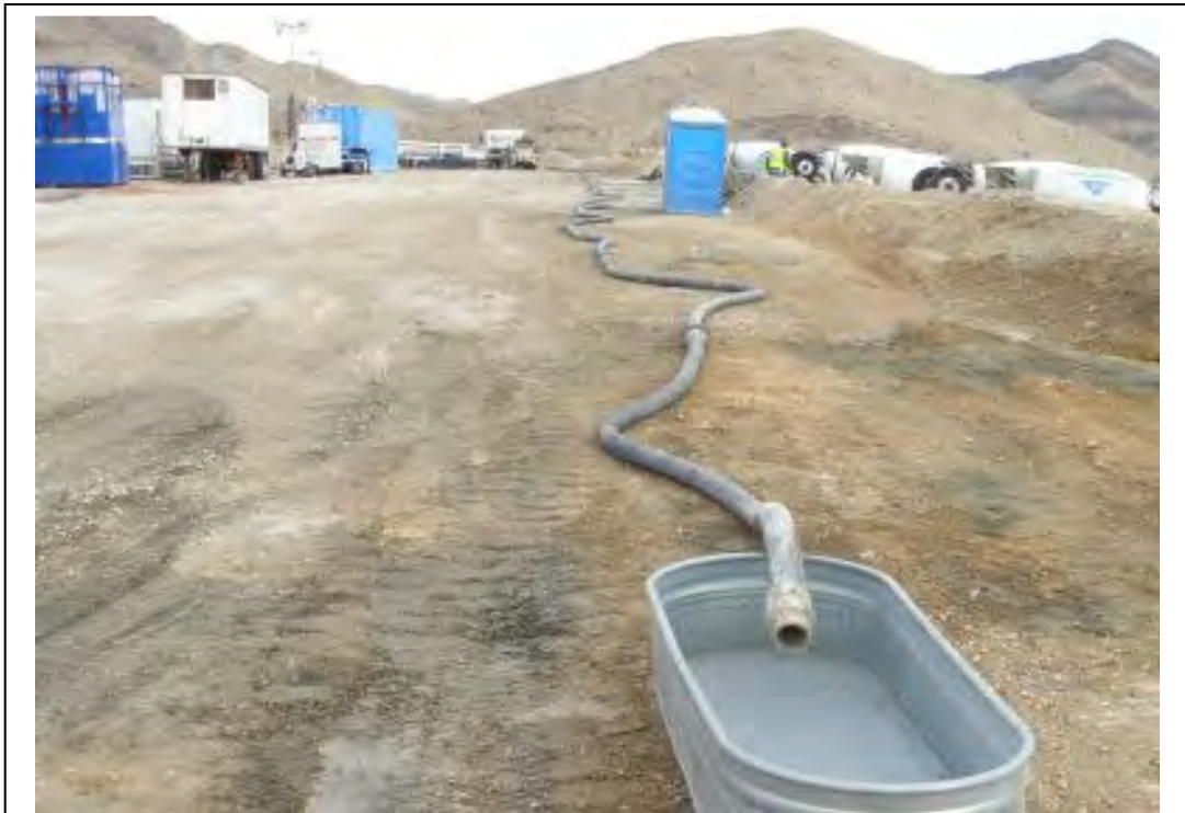
Figure 6.14: Pumping test - set up of pipeline
