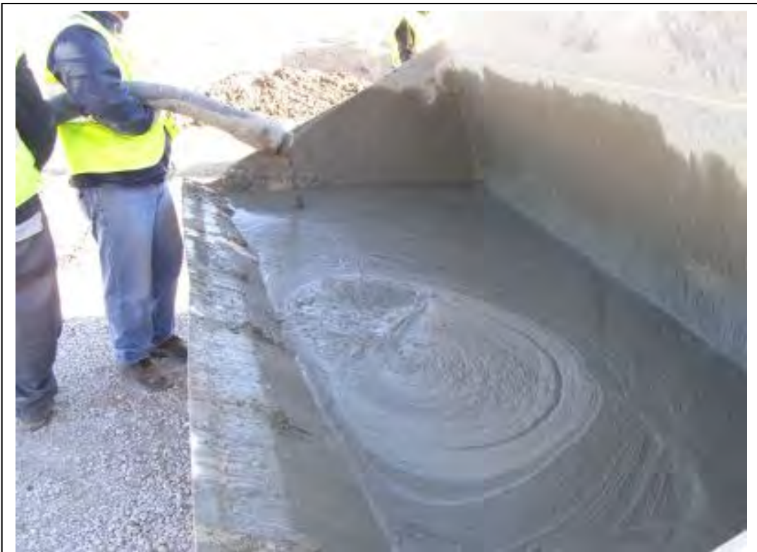
Figure 6.15: Pumping test - lubricating pipes with cement slurry
