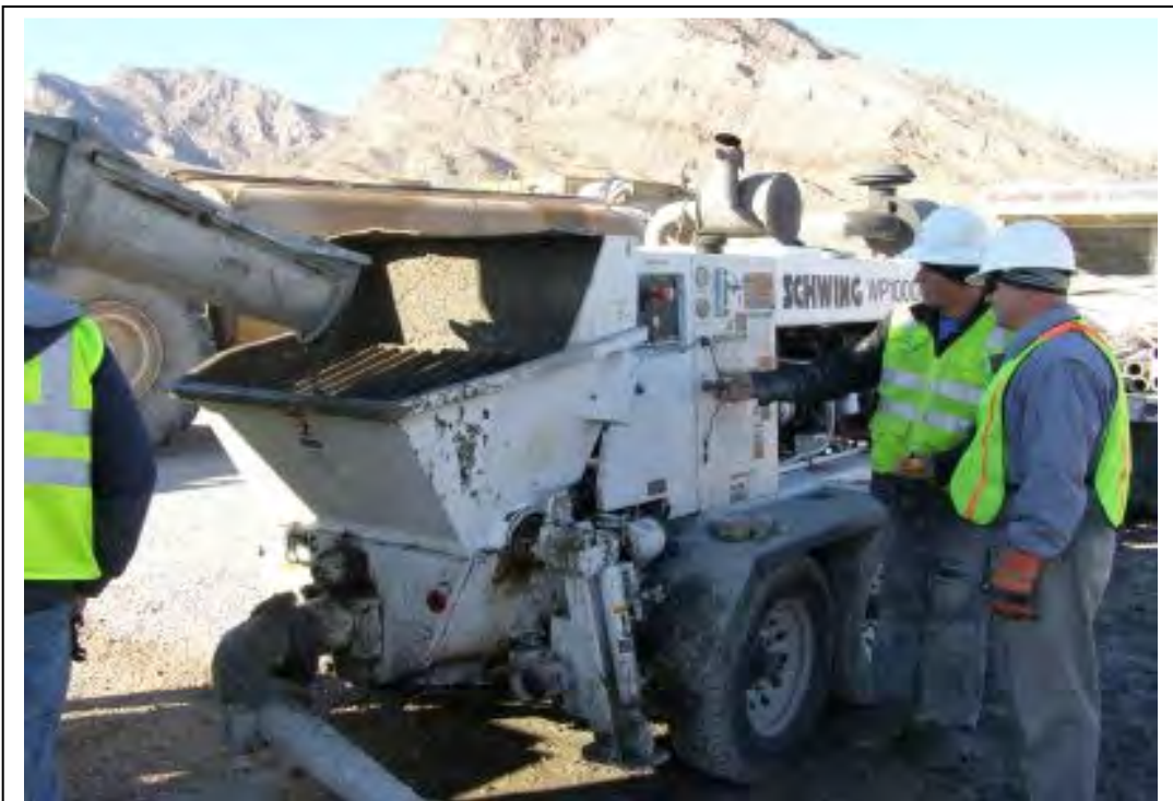
Figure 6.16: Pumping test - loading SCC in the receiving hopper
