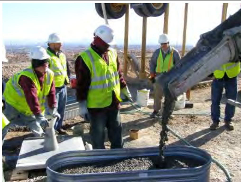
Figure 6.7a: Sample collection of SCC before pumping
