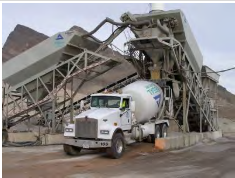
Figure 6.3: Loading of the concrete's dried ingredients
