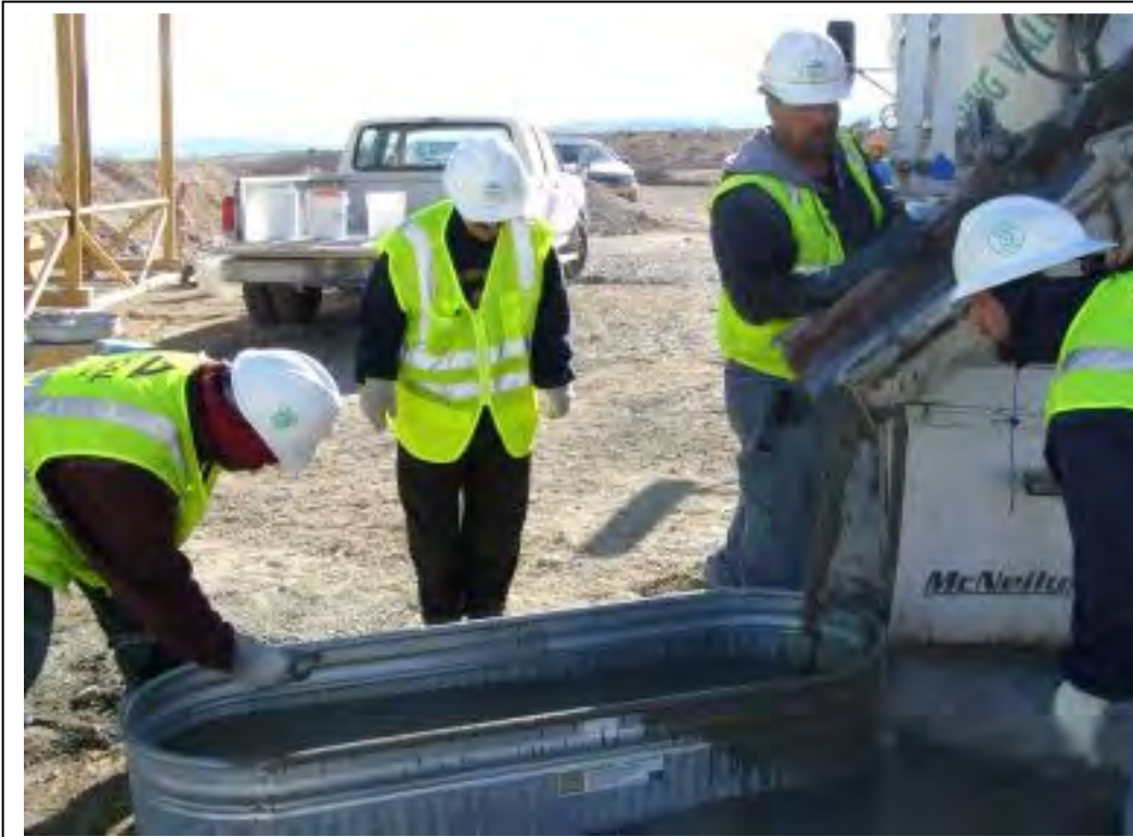
Figure 6.7b: Sample collection of SCC before pumping (continued)
