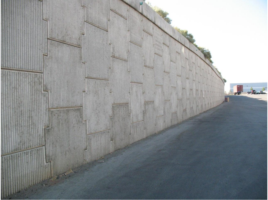
Figure 1. MSE Wall Located at South McCarran and I-80 (Contract #2957)
