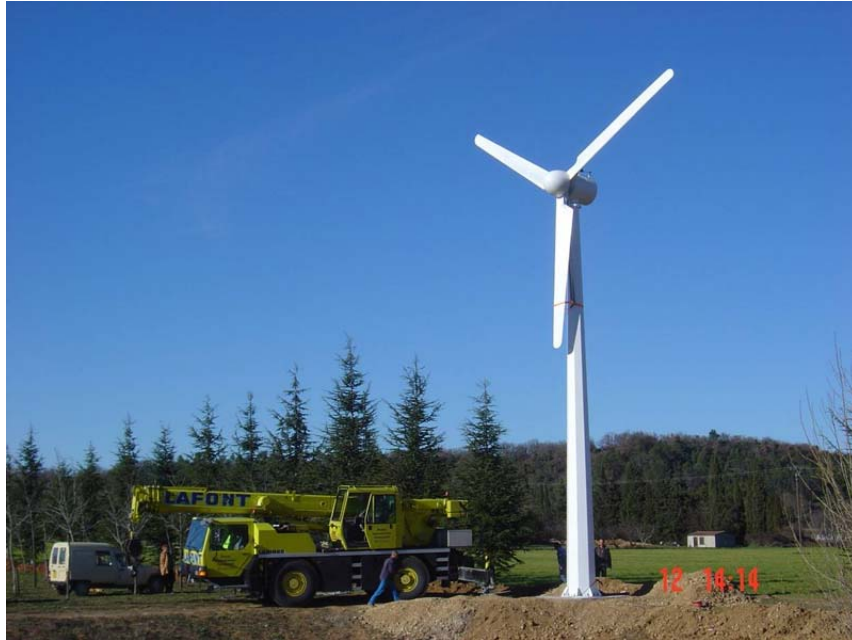
Fig 2.4 Image of a small wind turbine with 20 kW output power [9]
