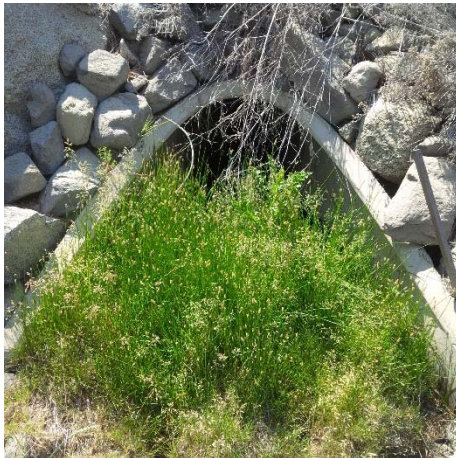
These photos indicate outlets for which maintenance is required.
