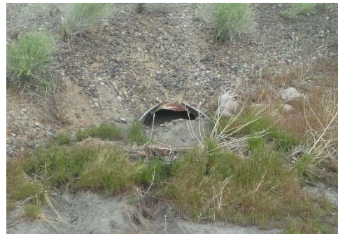
These photos indicate outlets for which maintenance is required.
