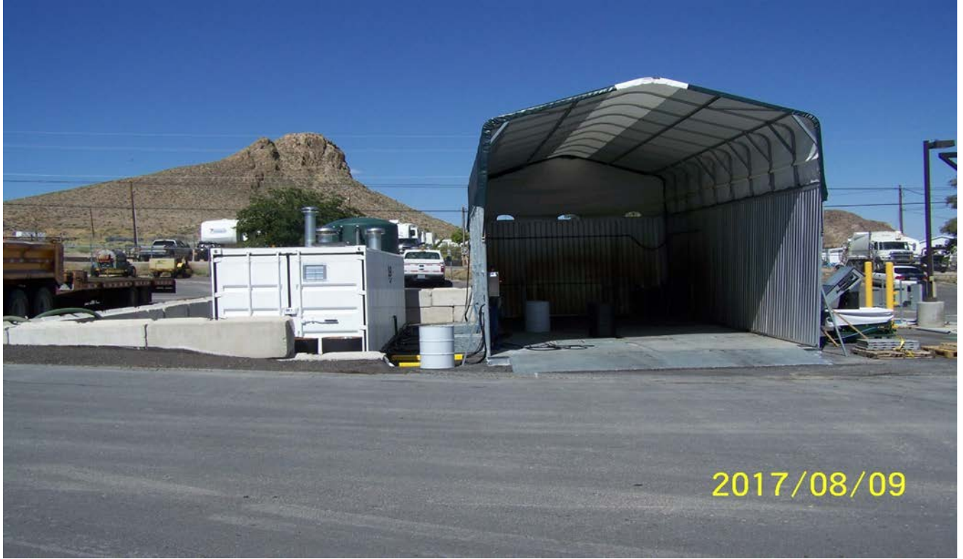
Self-contained equipment cleaning facility (Tonopah Station)
