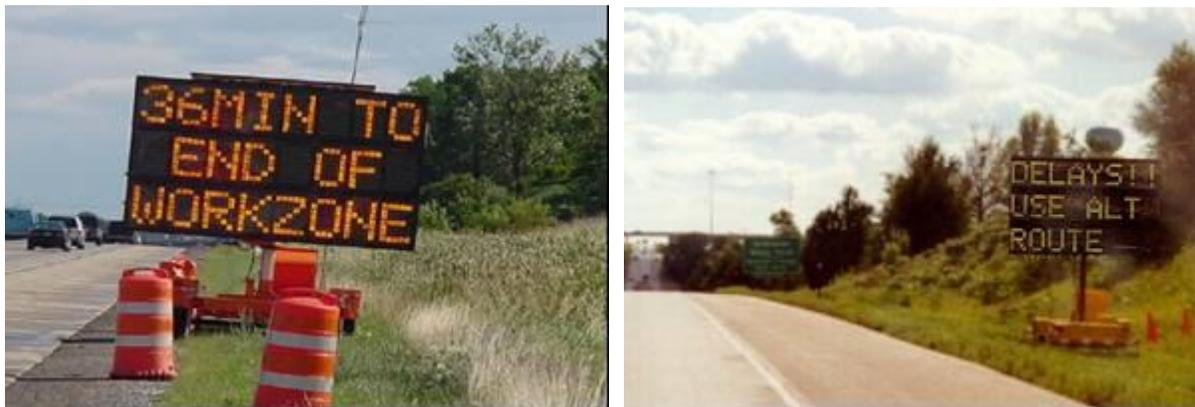
**Figure 1.2 Examples of Automatic Work Zone Information Systems for Disseminating Travel Time Information and Route Diversion**
