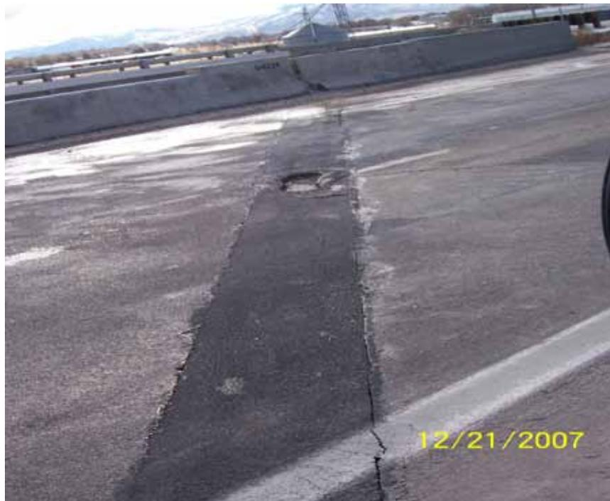
Figure 22 Bridge G-872 West Abutment (potholes, cracking)
