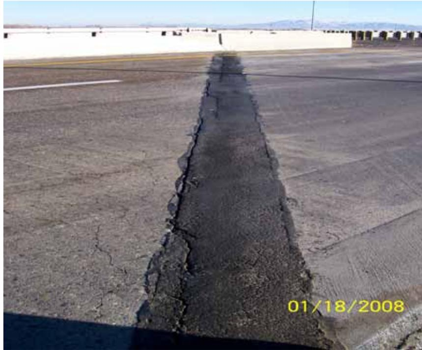
Figure 21 Bridge G-872 East Abutment (cracking, joint debonding)
