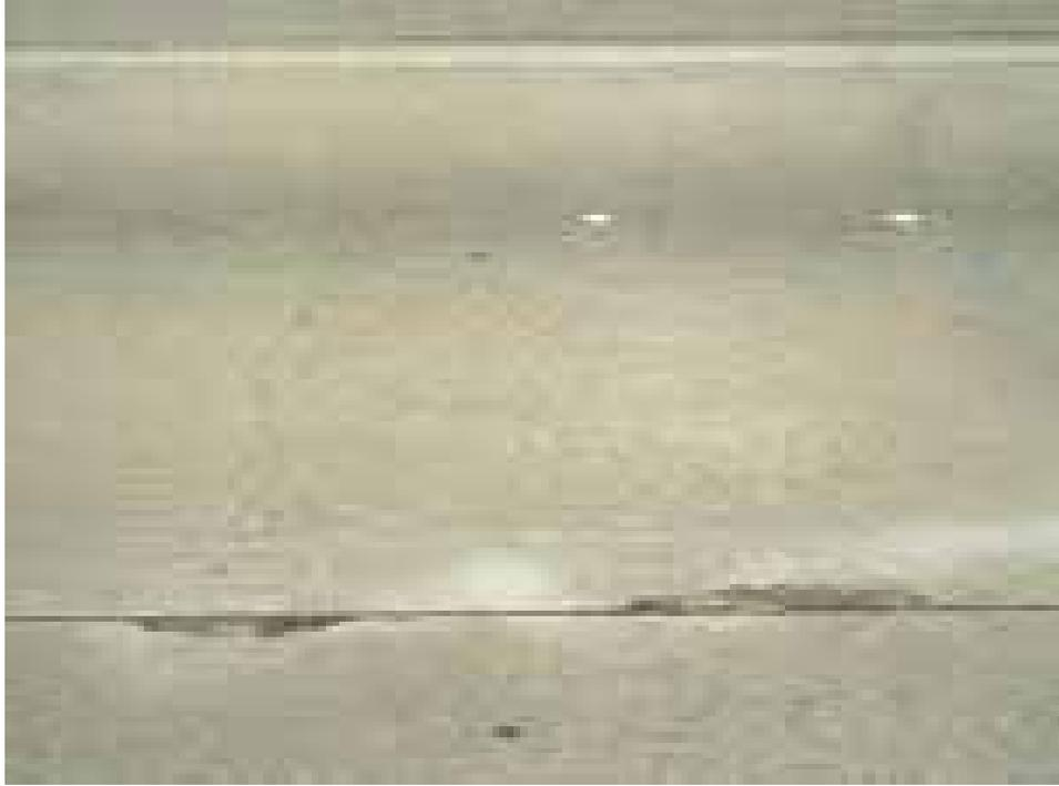
Figure 12 Spalling
