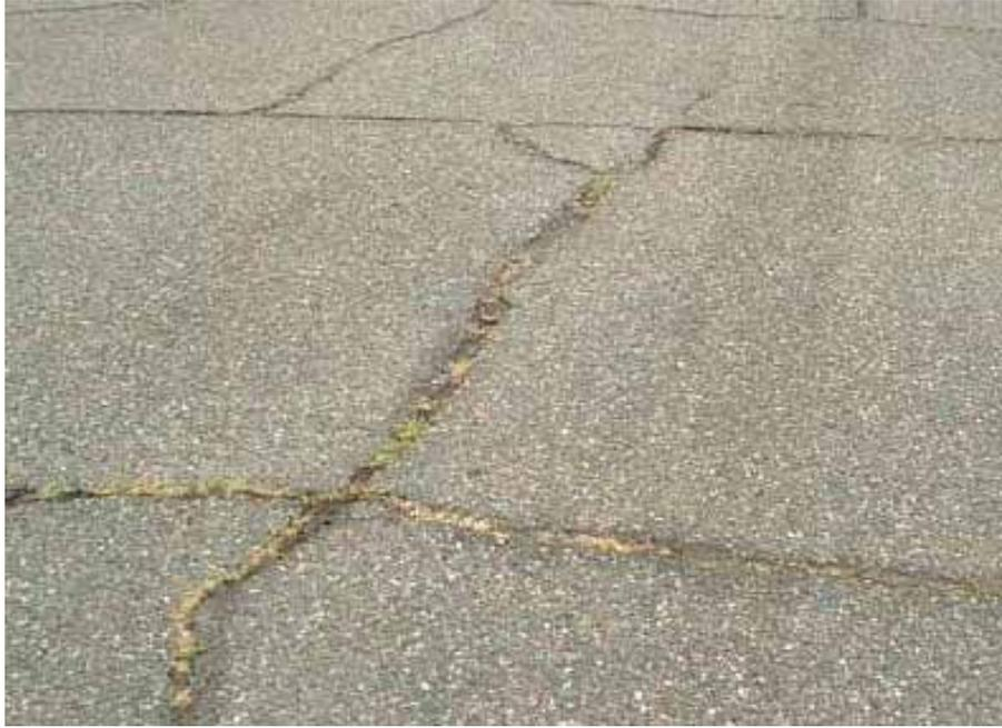
Figure 5 Reflective cracking
