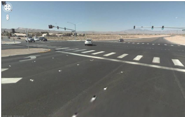
Figure 3-23 Picture of S. Dean Martin Dr/W Silverado Ranch Blvd Intersection
