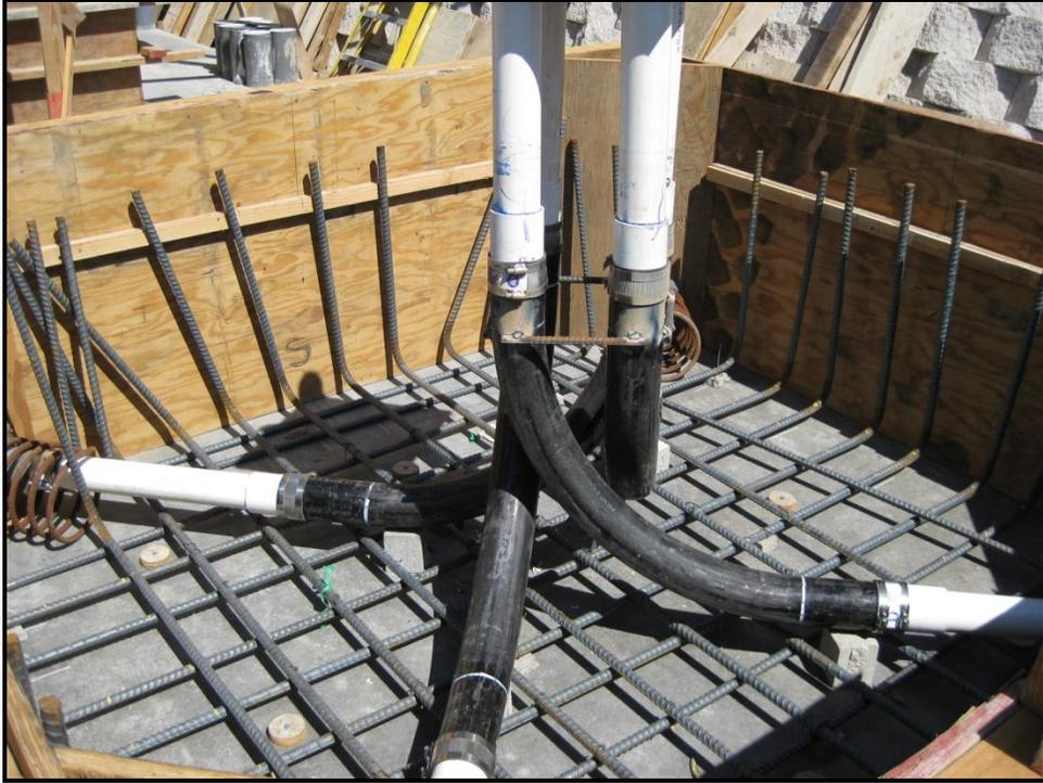
**Figure 2-11: Steel Pipes in Footing**
