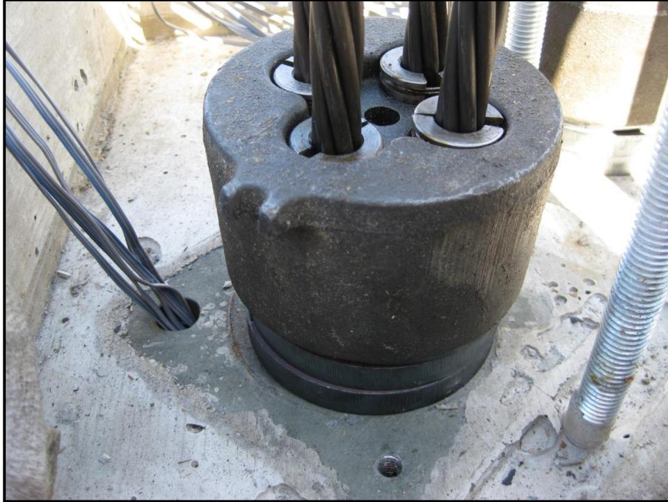
**Figure 2-19: Anchor Head on Shim Stack, Prior to Stressing**
