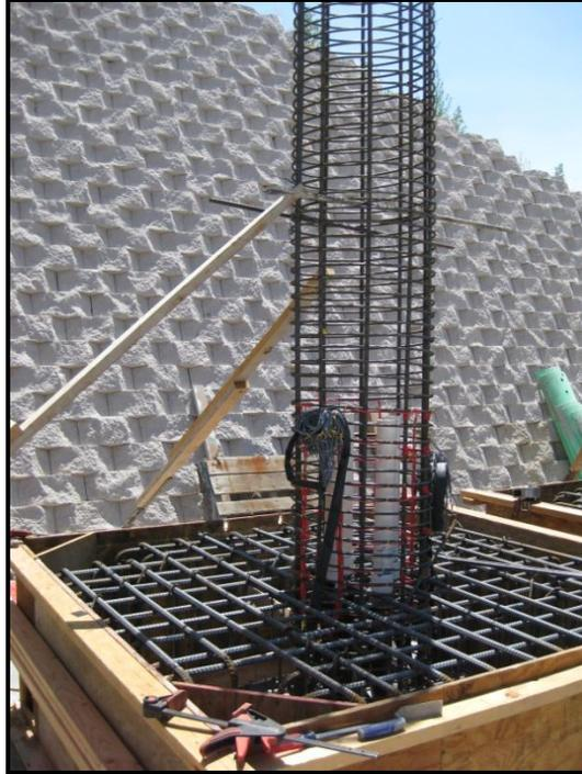
**Figure 2-13: Top Mat of Footing Reinforcement**
