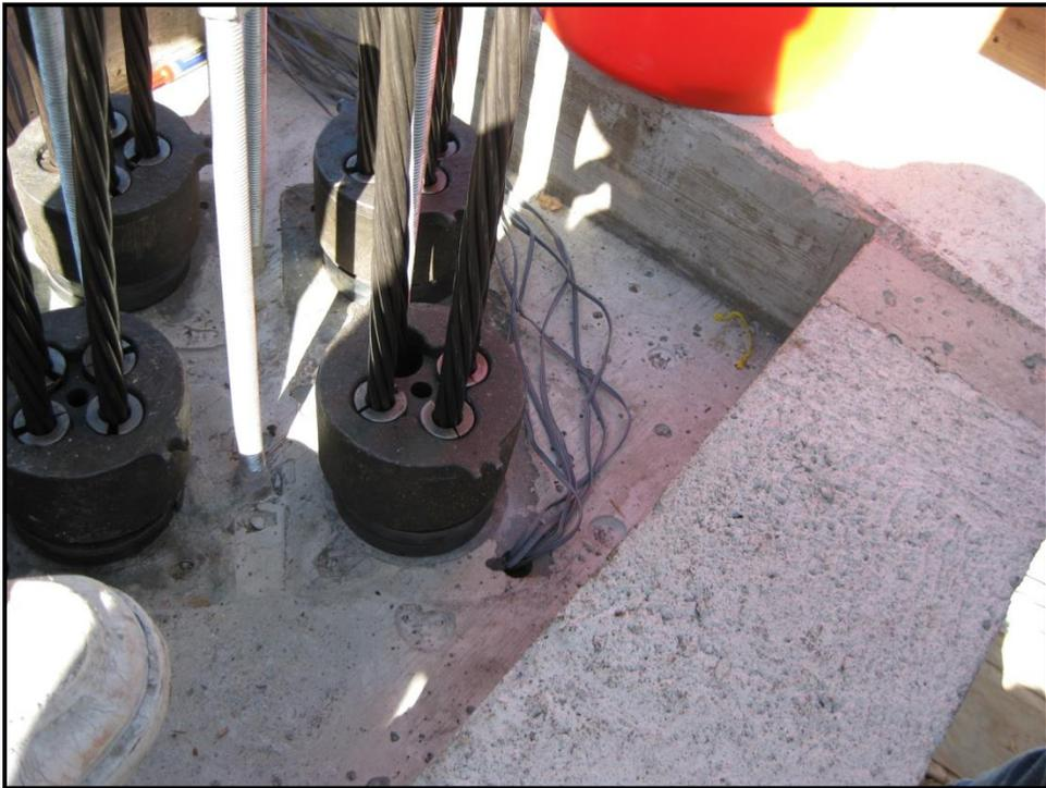
**Figure 3-5: Strain Gauge Wires Exiting Anchor Plate**
