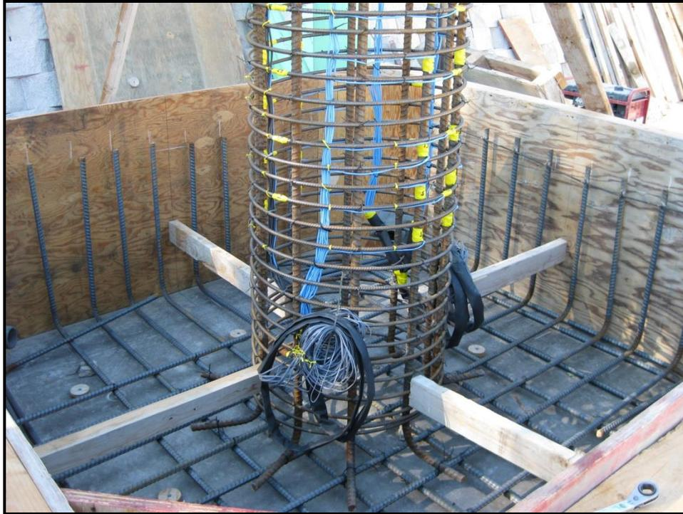
**Figure 3-2: Strain Gauges on Column Rebar Cage**
