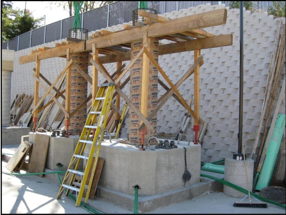
**Figure 2-15: Sonotube and Deck**
