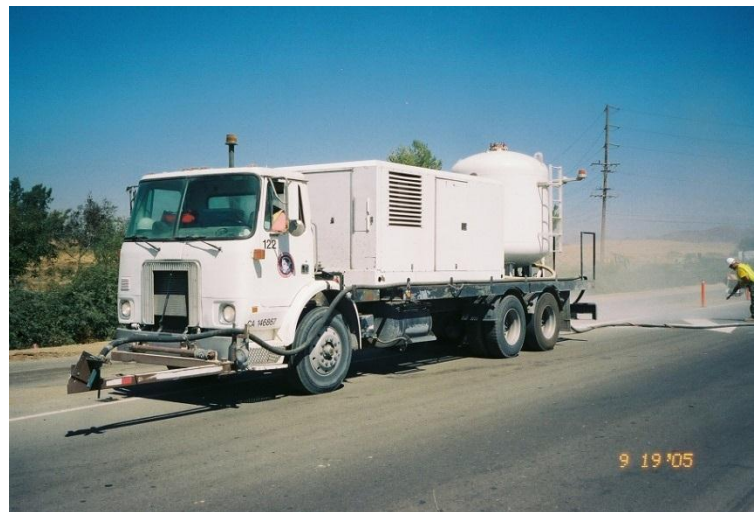
Fig.3 Sand blasting operations
