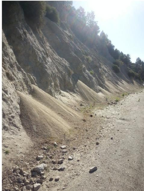
Figure 4.14. Dry ravel deposition cones along U.S. Highway 50
