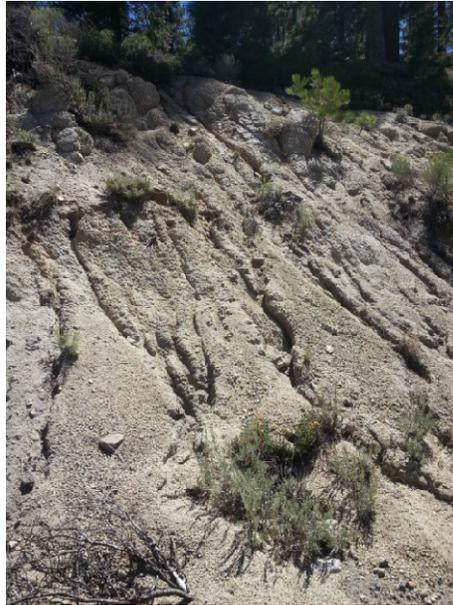
Figure 4.13. Rilling of cut slope along U.S. Highway 50
