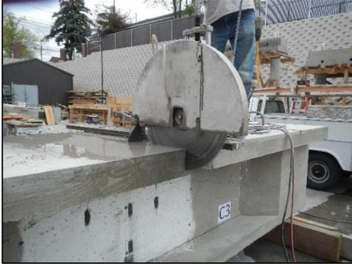
a) Cutting with a rotary saw.
