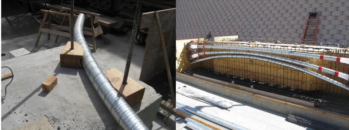
a) Technique used to bend steel ducts.      b) Steel ducts placed in the beam.
