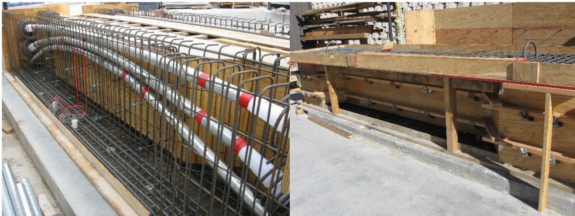
a) All shear reinforcement installed.      b) All forms and reinforcement installed.
