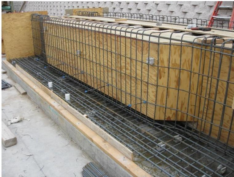
**Figure 2-36: One side of forms and shear reinforcement during construction.**
