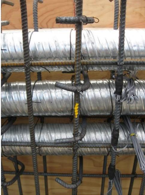
**Figure 2-40: Duct tie reinforcement bars installed in the beam.**
