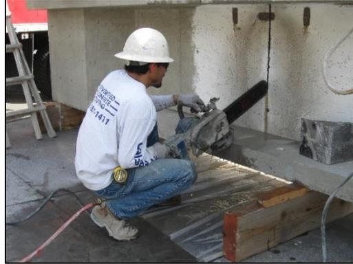
b) Cutting with a concrete chainsaw.
