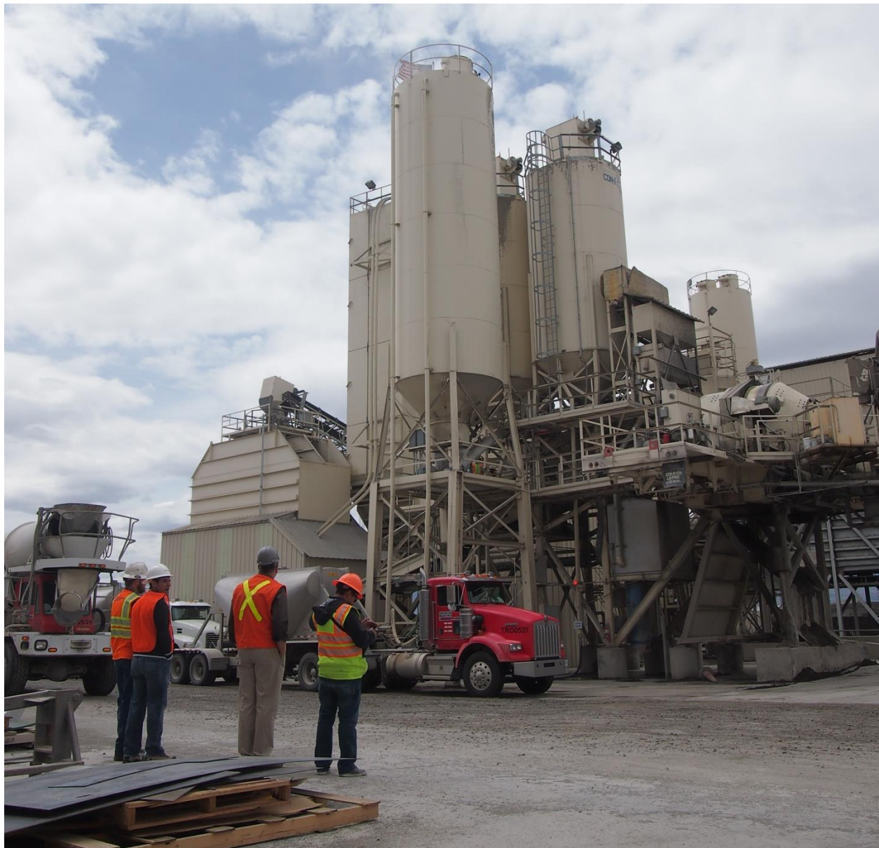
Figure 67 Central Mix Plant Setup for Trial Batch A.
