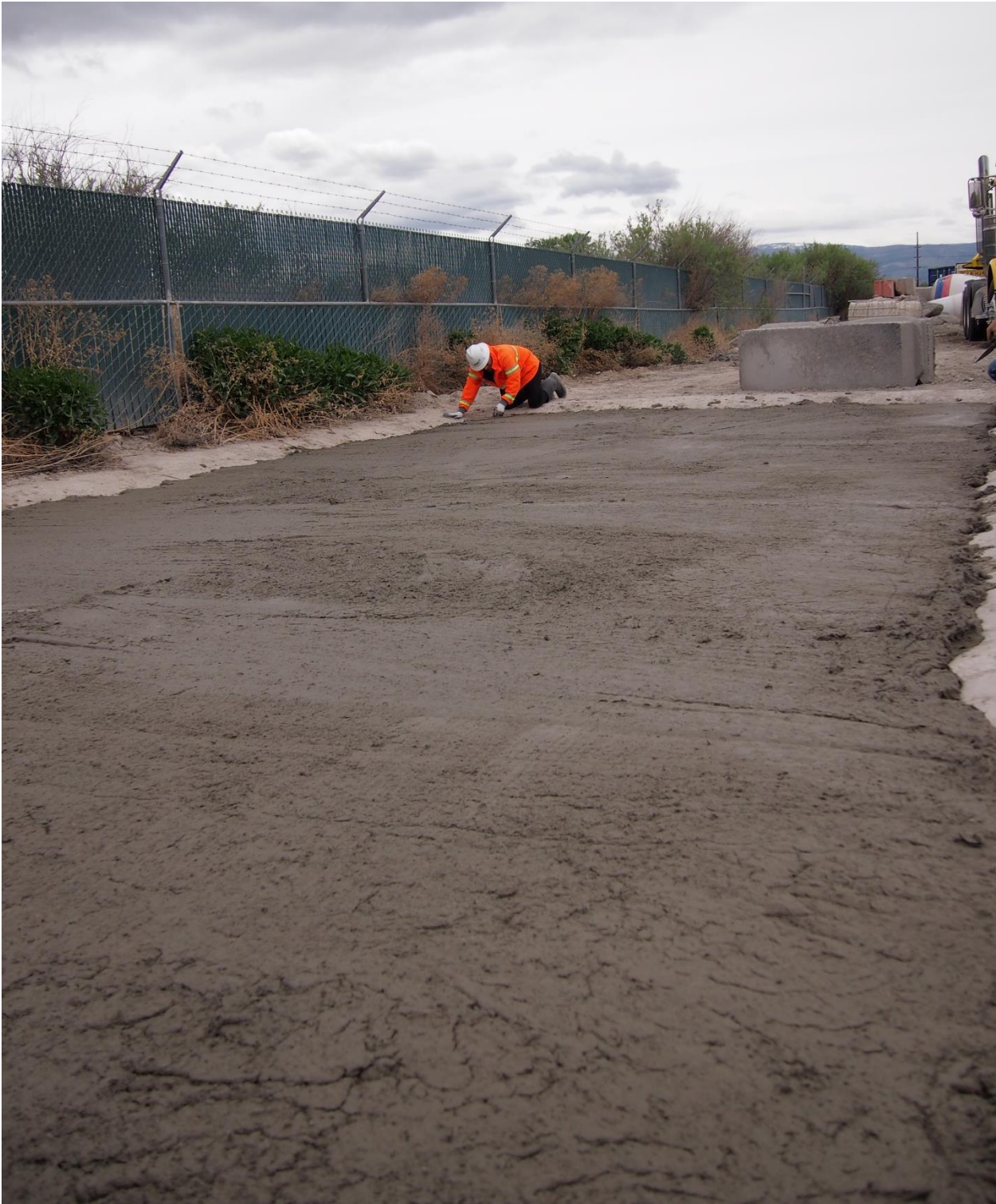
Figure 70 Completed Trial Slab from Trial Batch A.
