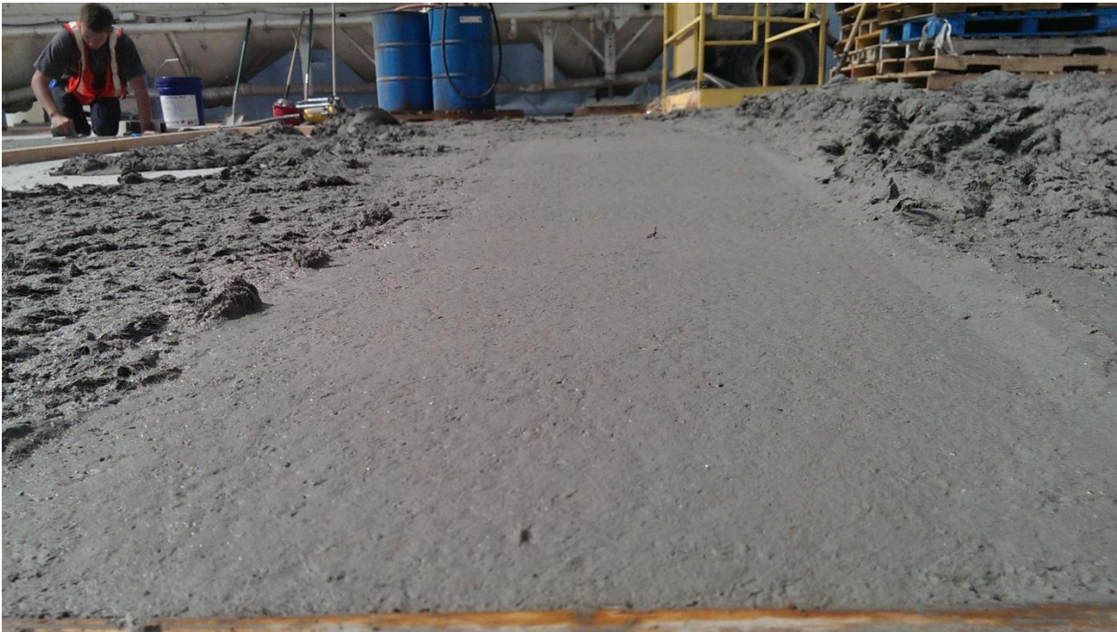
Figure 72 Completed Trial Slab from Trial Batch B.
