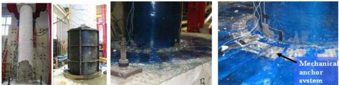
**Figure D.21** Restoration process for damaged column (Belarbi et al, 2008)
