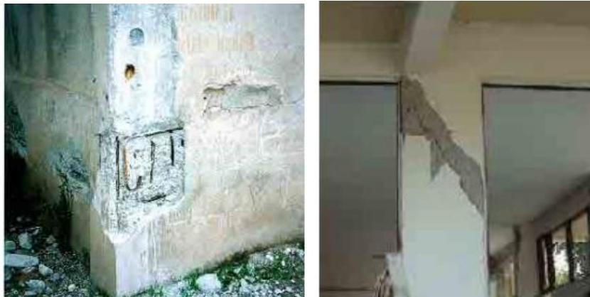
**Figure D.5** Damage state 4, extensive spalling and reinforcement exposure, but no buckling. (Kaminosono et al, 2002)
