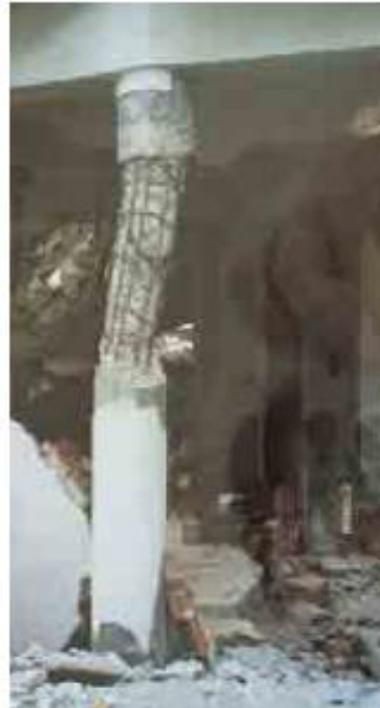
**Figure D.7** Damage state 5, fracture and buckling of reinforcement and collapse (Kaminosono et al, 2002)
