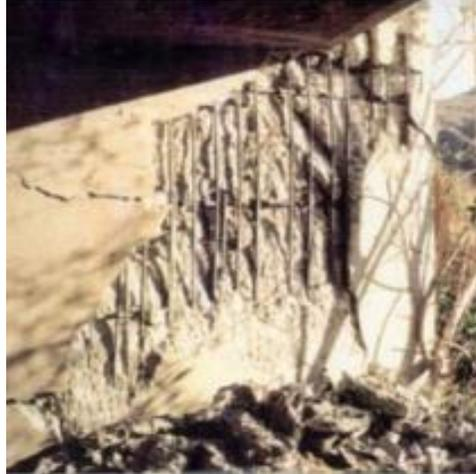
**Figure D.16** Abutment Damage State 6 (Saini et al, 2013)
