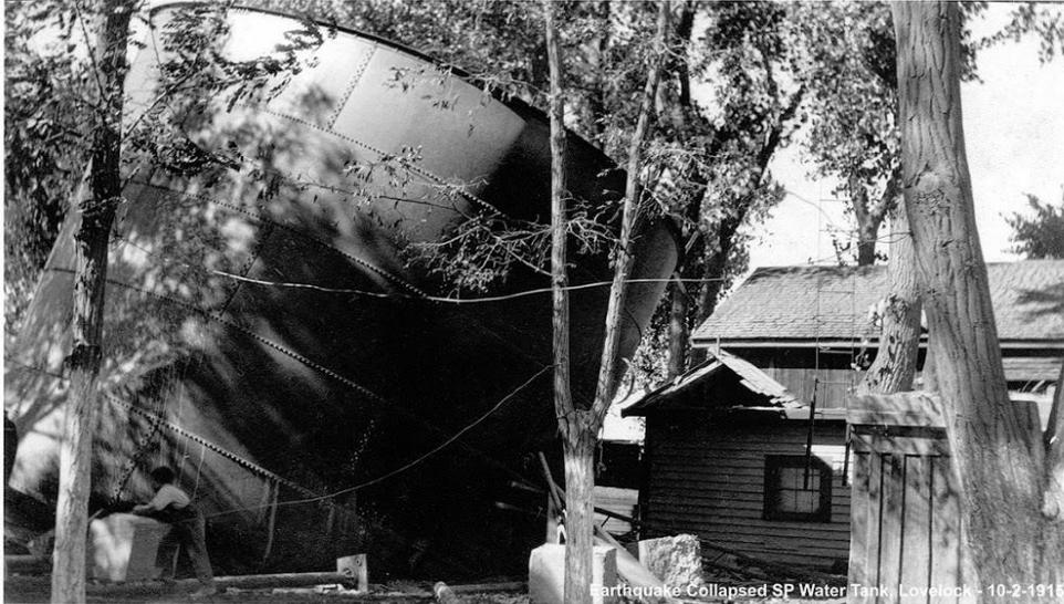
**Figure 2.1** Southern Pacific water tank in Lovelock, Nevada, damaged by ground motions of the 1915 Pleasant Valley M7.3 earthquake. Lovelock is approximately 60 km from the nearest part of the surface rupture. (photo source: <http://www.nbmng.unr.edu/Geohazards/Earthquakes/1915centennial.html>, accessed 10/21/2015; used with permission)
