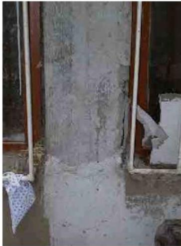
**Figure D.1** damage state 2, spalling of corner cover concrete (Kaminosono et al, 2002)
