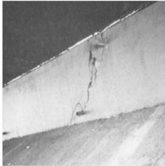
**Figure D.13** Abutment Damage State 2 (Saini et al, 2013)
