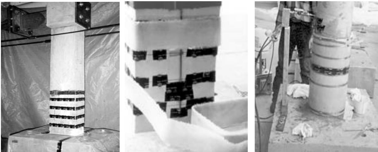
**Figure D.18** Repair process for columns (Saadatmanesh et al, 1997)
