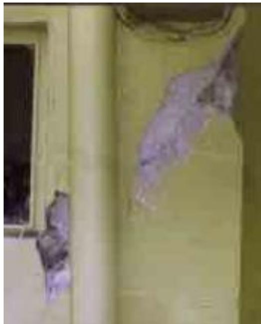
**Figure D.3** Damage state 3, wider shear cracking and local crush at top corner (Kaminosono et al, 2002)
