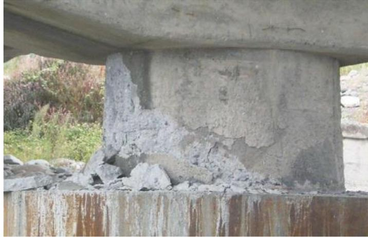
**Figure D.19** Shear damaged bridge Column (Li et al, 2003)
