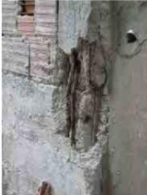
**Figure D.6** Damage state 4, massive spalling and exposure of reinforcement and minor buckling (Kaminosono et al, 2002)
