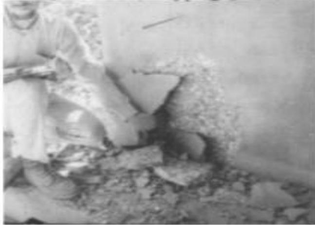
**Figure D.14** Abutment Damage State 3 (Saini et al, 2013)
