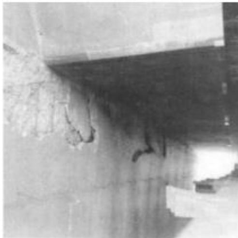
**Figure D.15** Abutment Damage State 4 (Saini et al, 2013)
