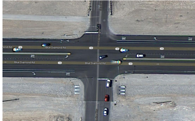
Figure 5.3 Intersection Picture at Blue Diamond Road and South El Capitan Way
