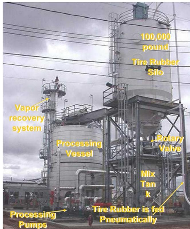
**Figure 2.10. Terminal Blending Process of Rubberized Binder (29)**
