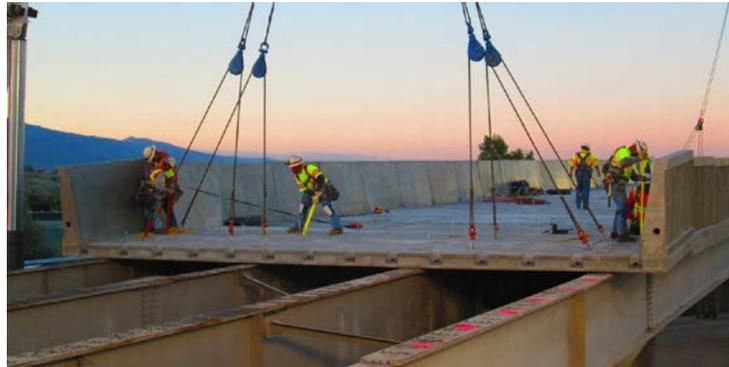
Figure 2.44: Deck placement of Utah ramp (Scoles et al, 2014)
