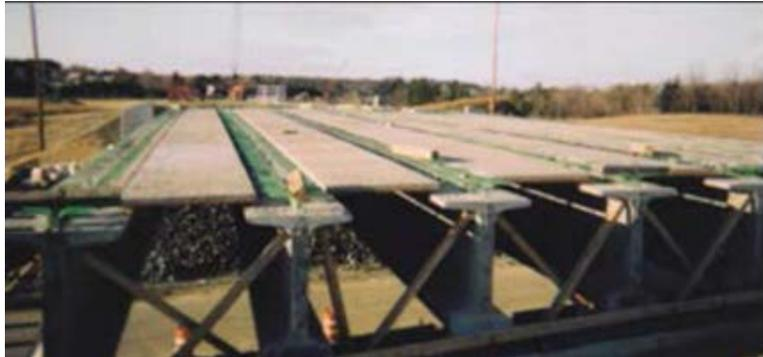
Figure 2.2: Partial depth concrete deck (Culmo, 2011)
