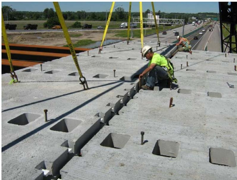
Figure 2.1: Full depth precast concrete deck (Culmo, 2011)
