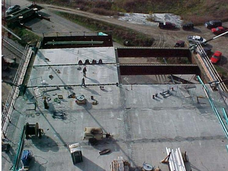
Figure 2.15: Longitudinal cast-in-place joint (Badie and Tadros, 2008)
